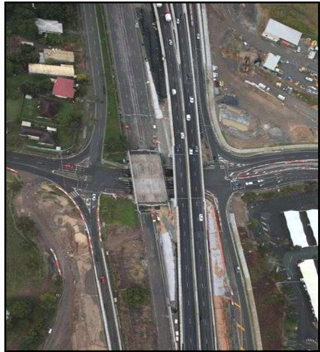
The old Mine Street bridges ready to be removed
