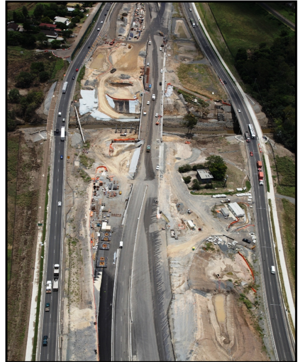
Construction works at Six Mile Creek
