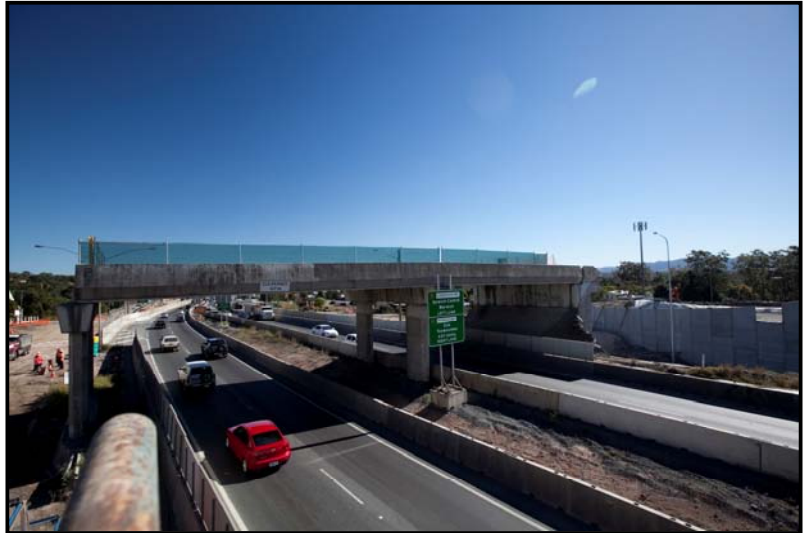
The old Tessman Street Bridge ready for demolition
