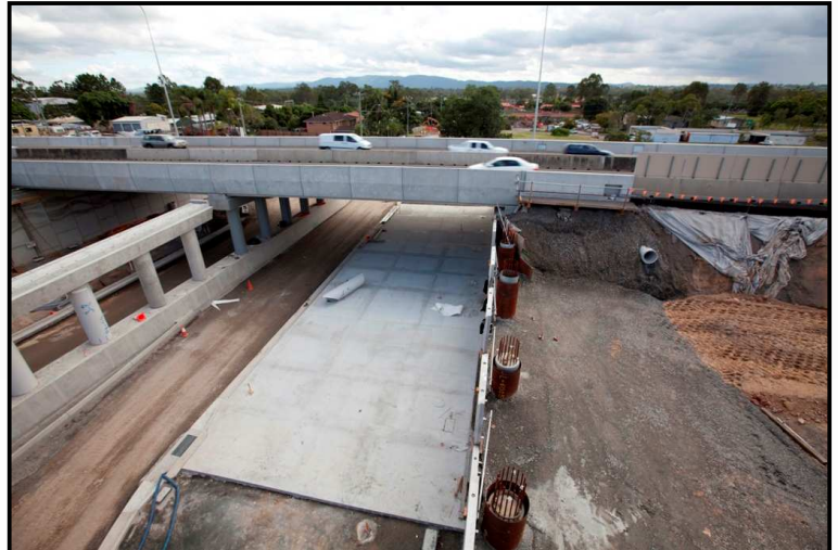
The Endeavour Road connection at Riverview is taking shape.
