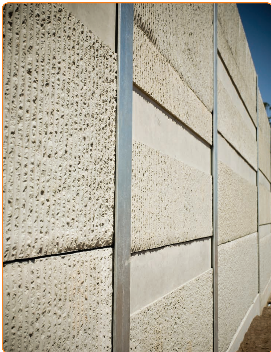
Noise barriers work by interrupting the path of sound waves.
