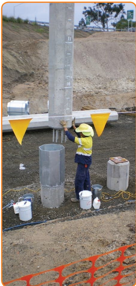
Pitching a pile into a pre-bored hole.
