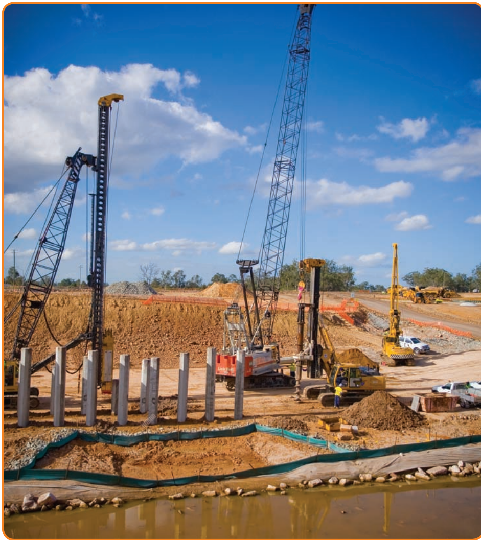
Piling for bridge structures over local waterways.
