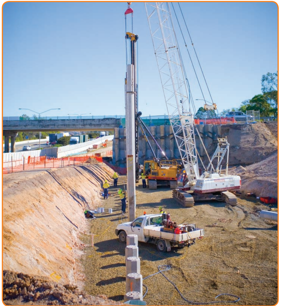
Piling within the Centenary Highway Interchange.
