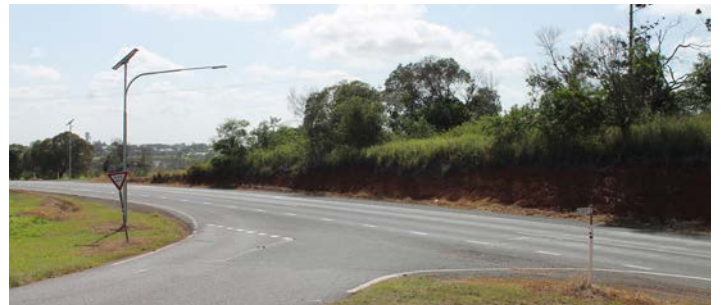
Planning is progressing to upgrade the Old Creek Road (south) intersection
