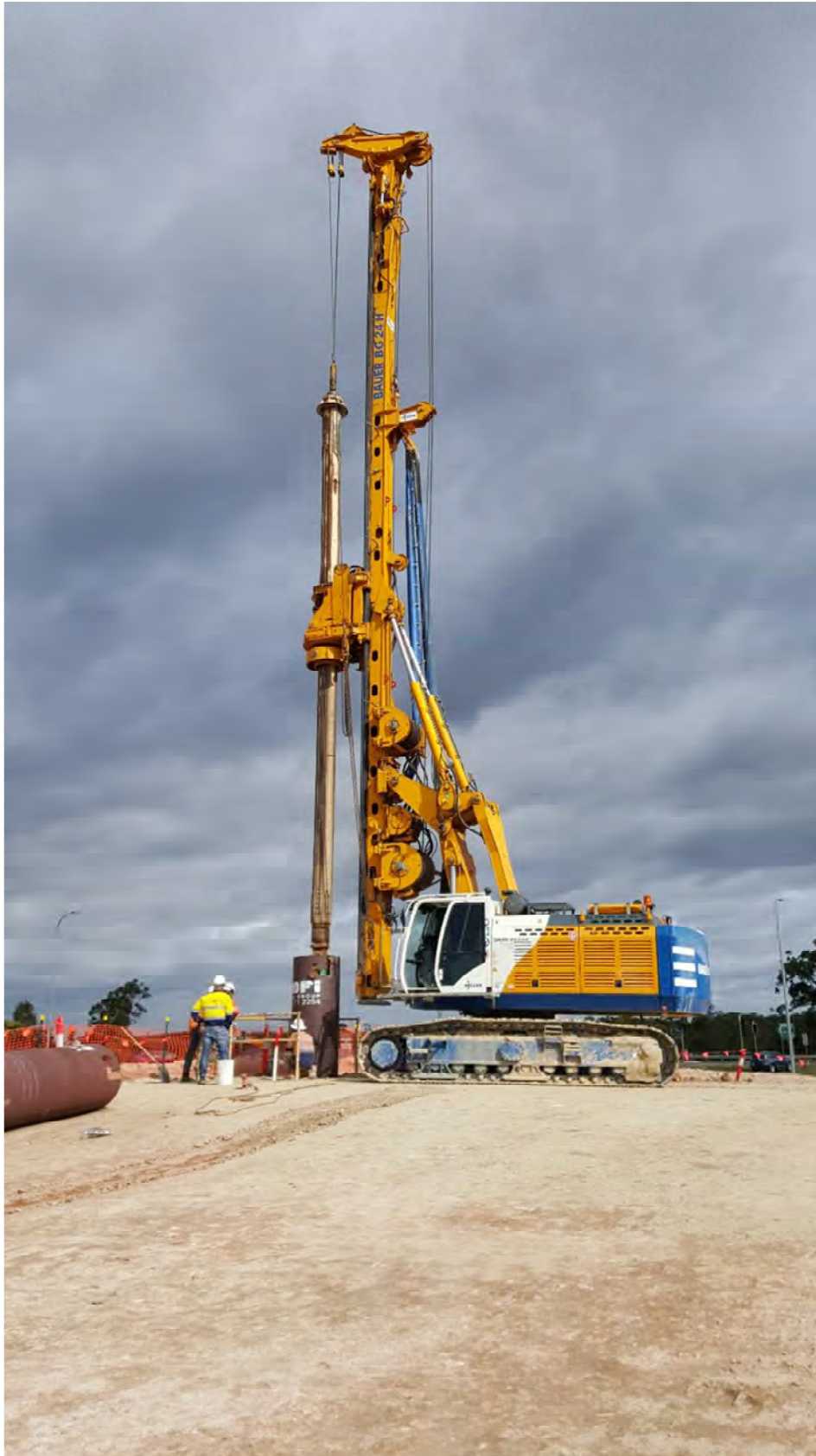
Piling rig – undertaking piling activities for the new six-lane bridge
