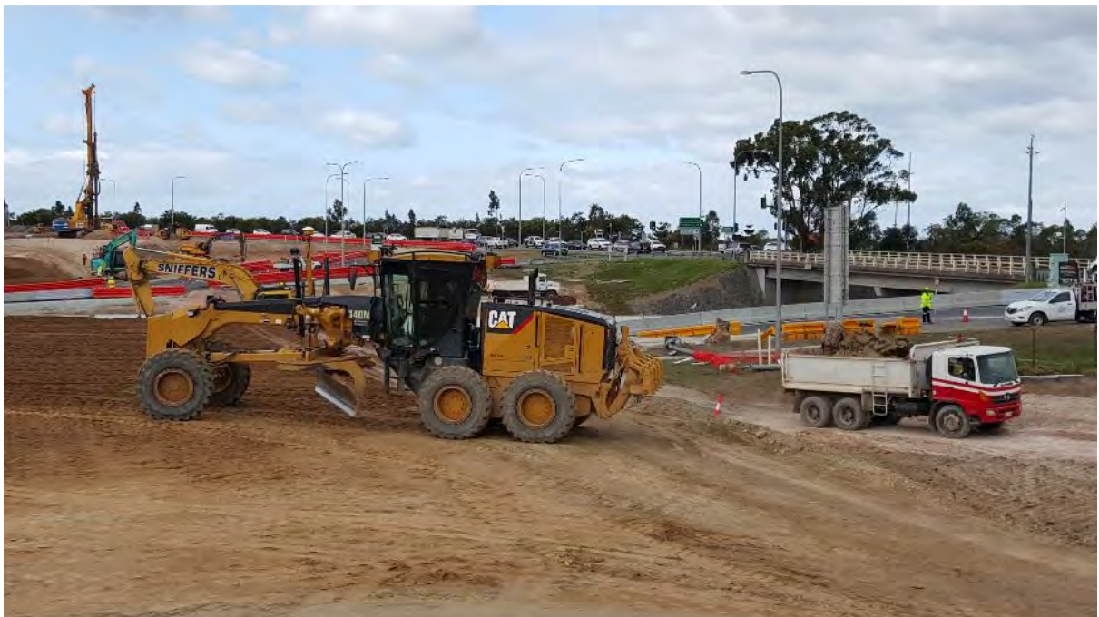
Activities onsite – bulk earthworks and bridge piling
