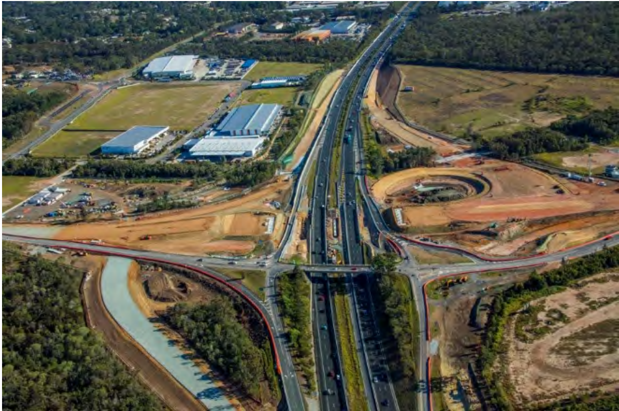
Boundary Road/Bruce Highway interchange upgrade – looking northbound
