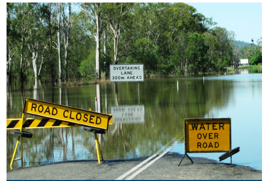
Bruce Highway flooding at Tiaro (Chinaman Creek Bridge), 2013
