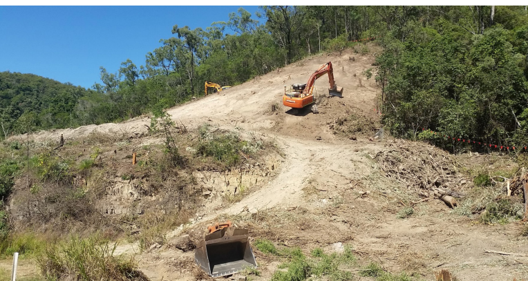
Clearing and excavation works undertaken in May 2016.
