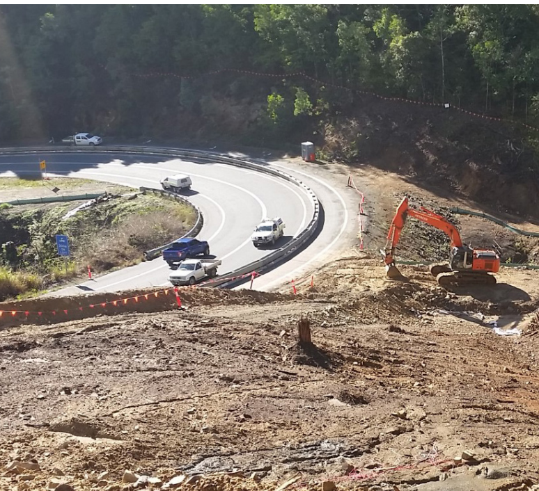
Earthworks activities undertaken in June 2016.
