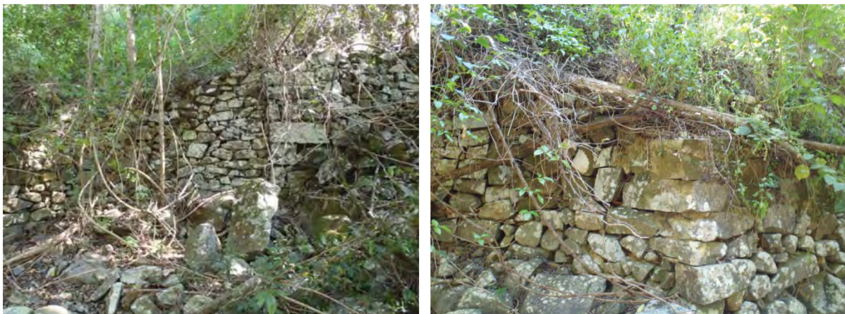
Plate 2 & 3: Rock wall abutments of old Cobb & Co. route
