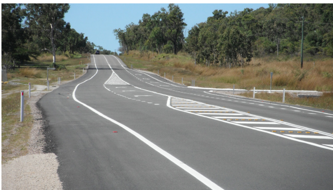
Dedicated right and left turning lane combination
