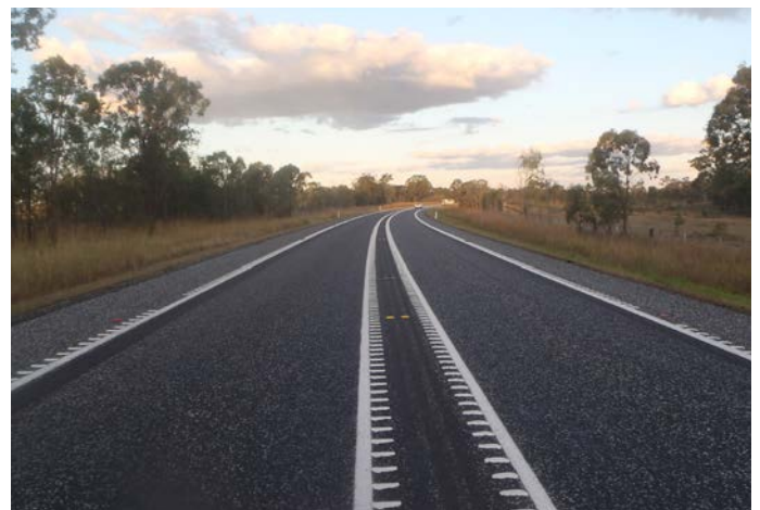
Caption: Wide centre line treatment with audio tactile line marking
