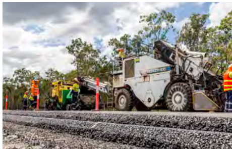
EME2 asphalt being laid
