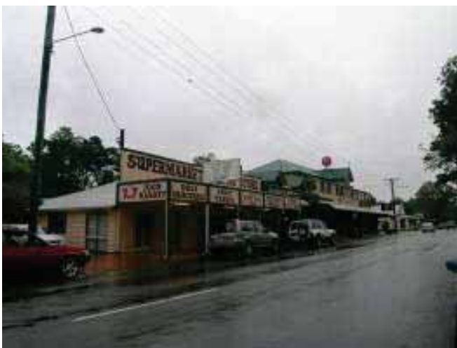
Figure 7.2.4a: View to Cribb Street facing north west
