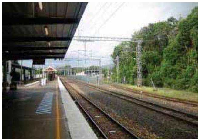
Figure 7.6.5a: View south of Nambour Station
