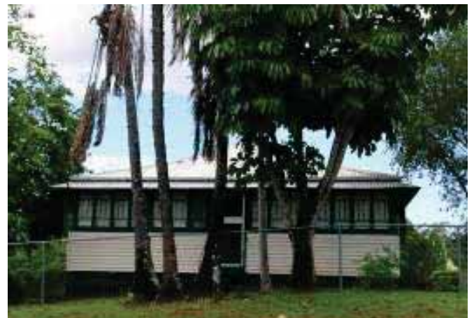
Figure 7.5.4c View to bungalow Chevallum Road from west.
