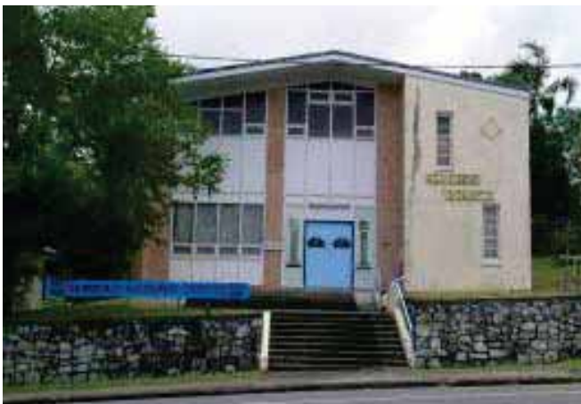
Figure 7.6.4f: View to Masonic Lodge, Blackall Terrace, Nambour
