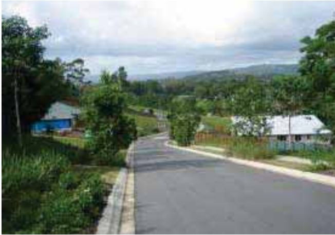
Figure 7.6.5c: View west across the new Rangebrook Estate to the existing railway corridor (in cutting) and bridge.
