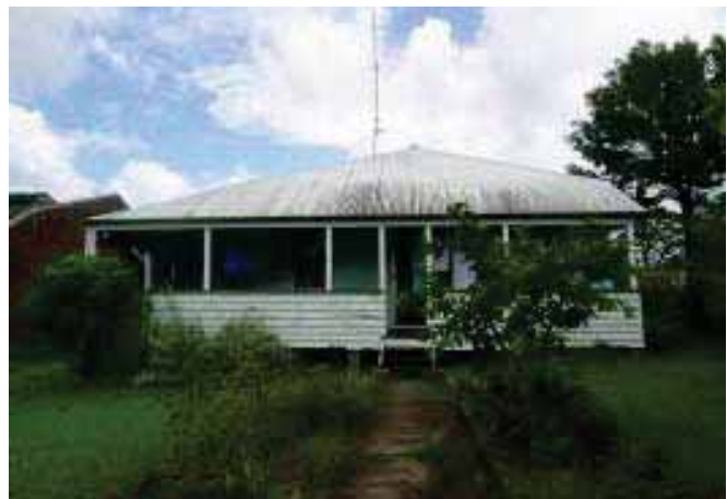
Figure 7.6.4c: View to 19 Mill Street from west
