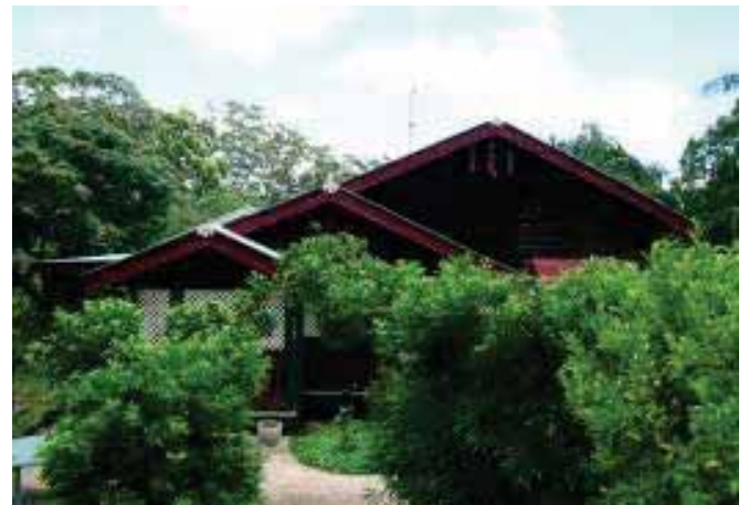
Figure 7.5.4b: View to multi gabled house, Chevallum Road from east.
