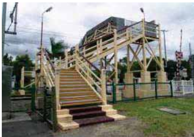
Figure 7.3.4a: Mooloolah Rail Bridge.
