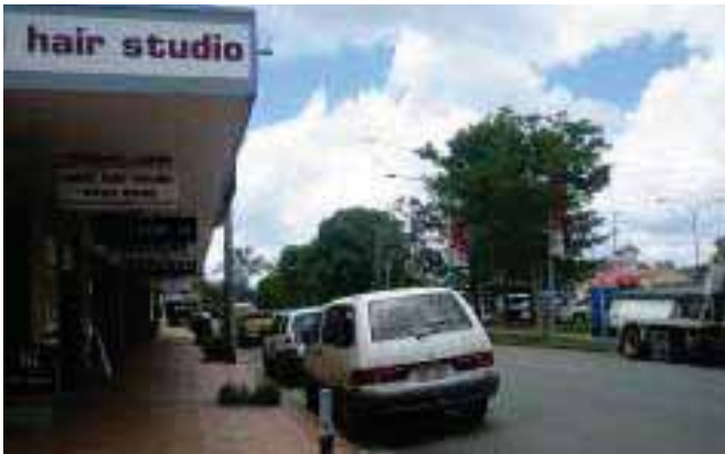
Figure 7.2.5a: View north along Cribb Street civic centre.
