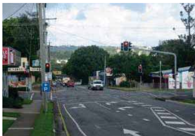
Figure 7.6.5b: View west along Arundell Avenue to the existing railway bridge.
