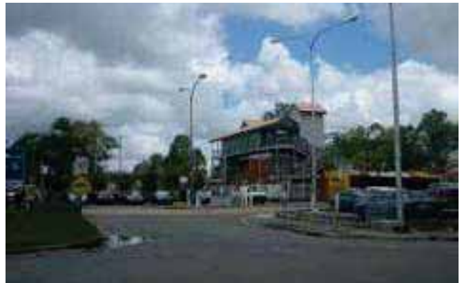
7.2.5d: View east from Cribb Street to Landsborough Railway Station & pedestrian overpass.
