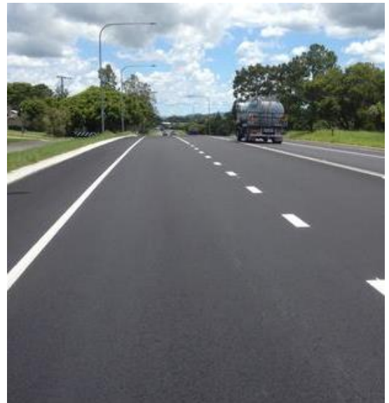
An example of asphalt surface
