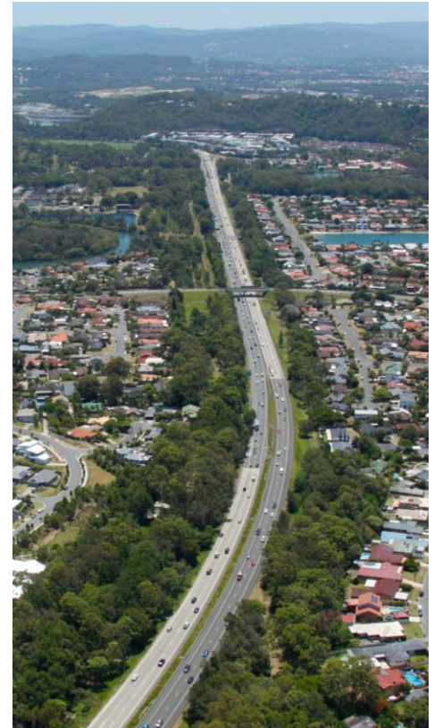
VL2T section of the M1 including the 19 th Avenue overpass
