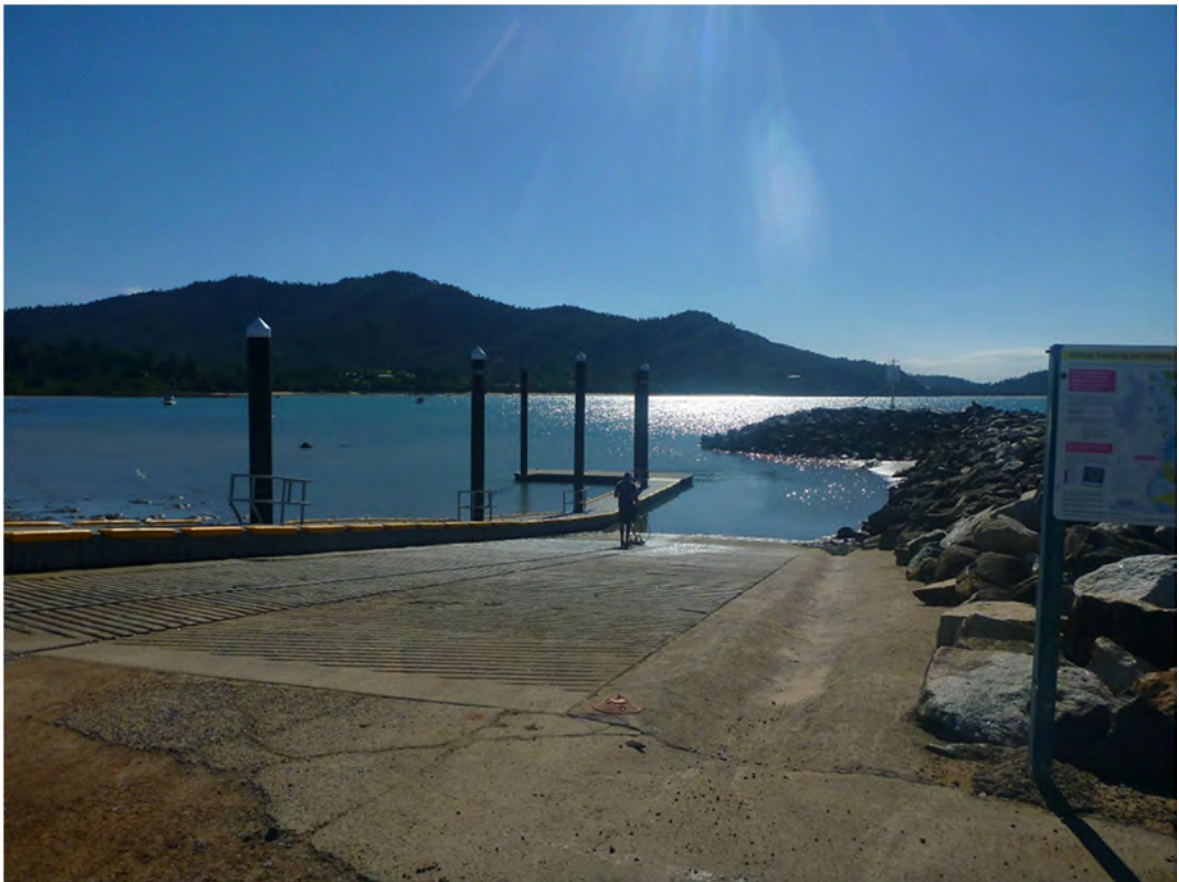
Figure 2-1 Clump Point Boat Ramp, Floating Walkway and Rock Breakwater
