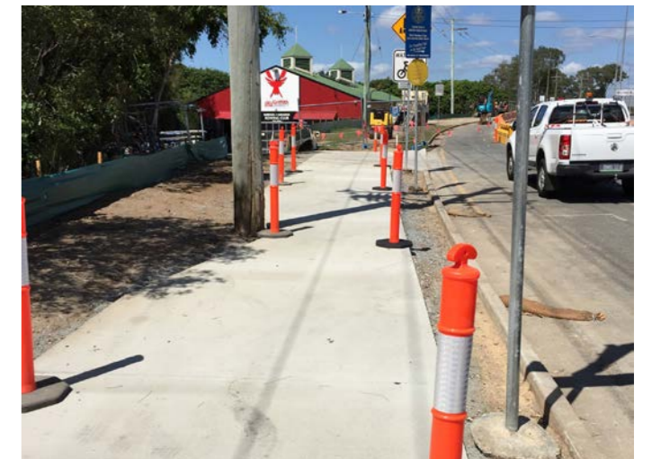
Construction of the off-road shared pedestrian and cycle pathway on Bundall Road.
