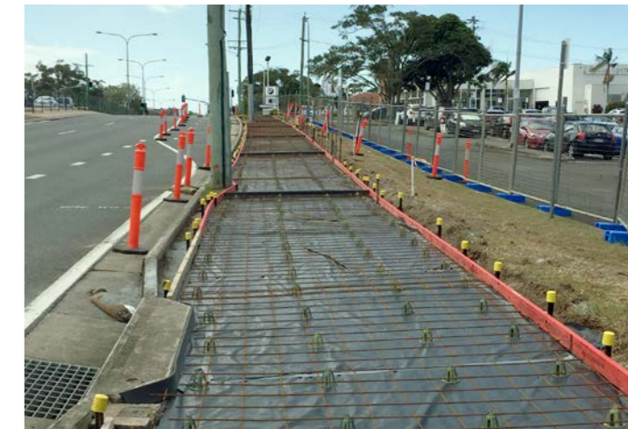
Footpath works on High Street
