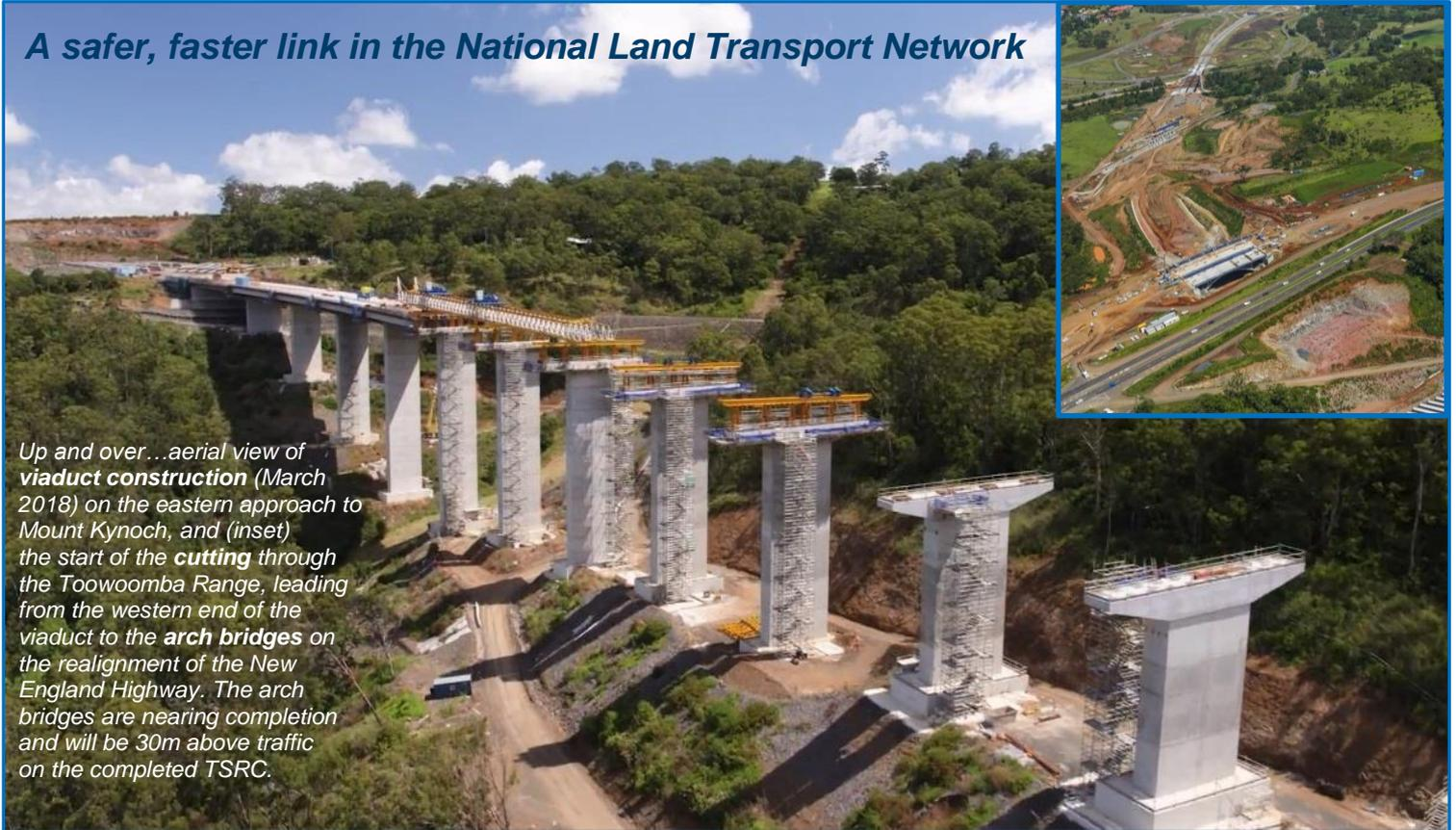
*Up and over... aerial view of viaduct construction (March 2018) on the eastern approach to Mount Kynoch, and (inset) the start of the cutting through the Toowoomba Range, leading from the western end of the viaduct to the arch bridges on the realignment of the New England Highway. The arch bridges are nearing completion and will be 30m above traffic on the completed TSRC.*
