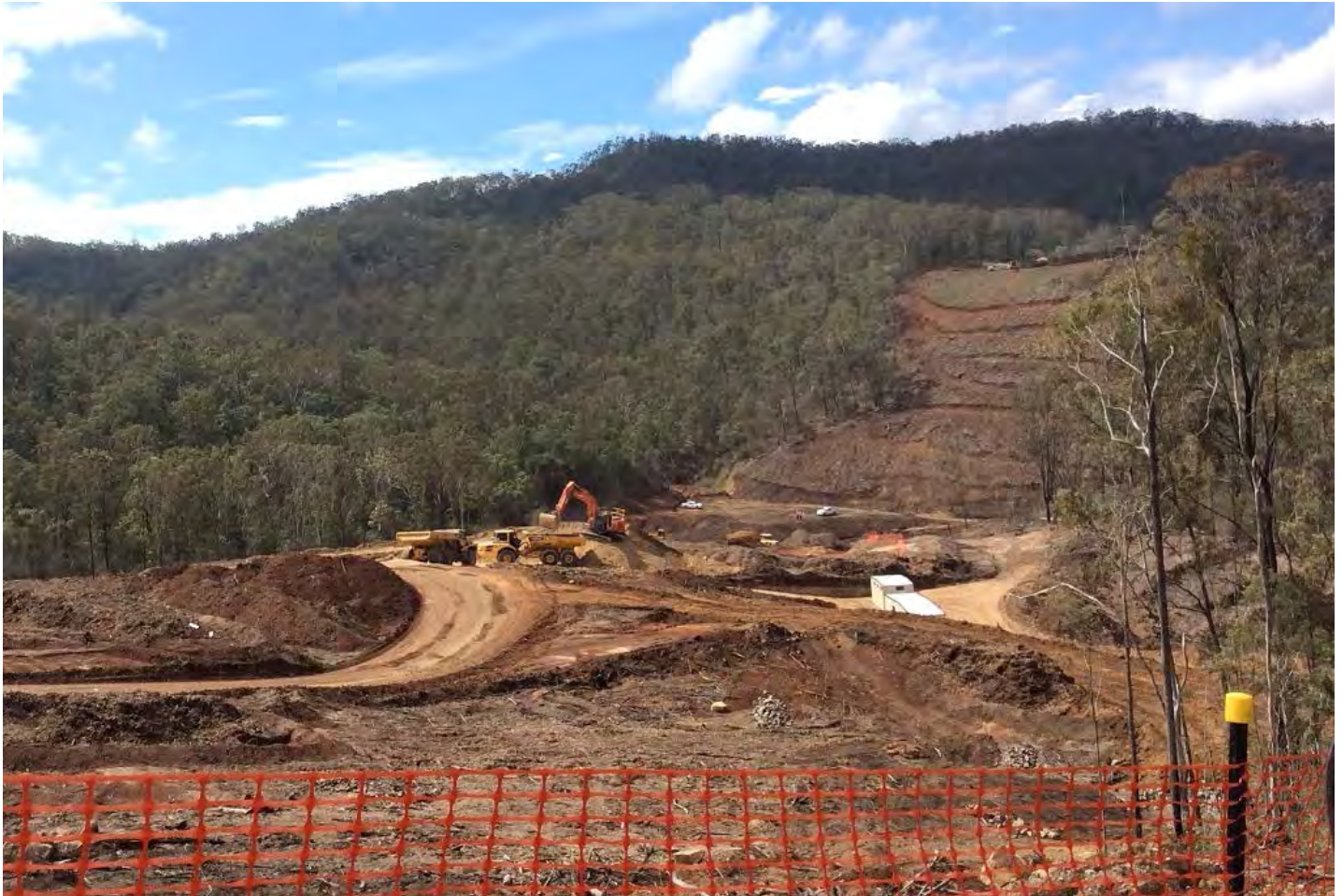
Excavation underway near Morleys Road underpass at Ballard, north-east of Toowoomba.
