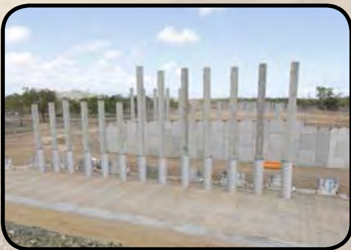
Bridge substructures at the northern interchange
