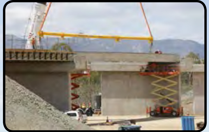
Placing bridge deck units on the Dalrymple Road Overpass
