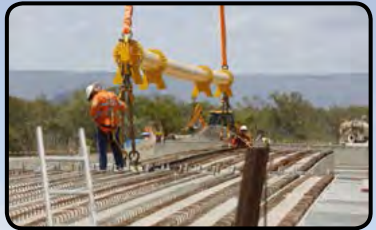
Securing bridge deck units in place
