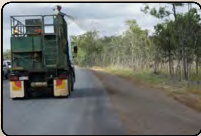
Spraying hydromulch to grass embankments
