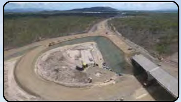
Aerial view of the Dalrymple Road Overpass
