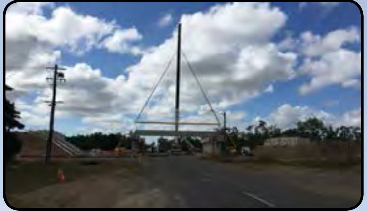
Lowering bridge deck units in place on Geaney Lane
