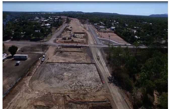
Geaney Lane overpass taking shape
