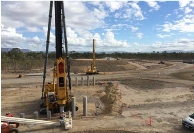
Pile driving on the Dalrymple Road interchange
