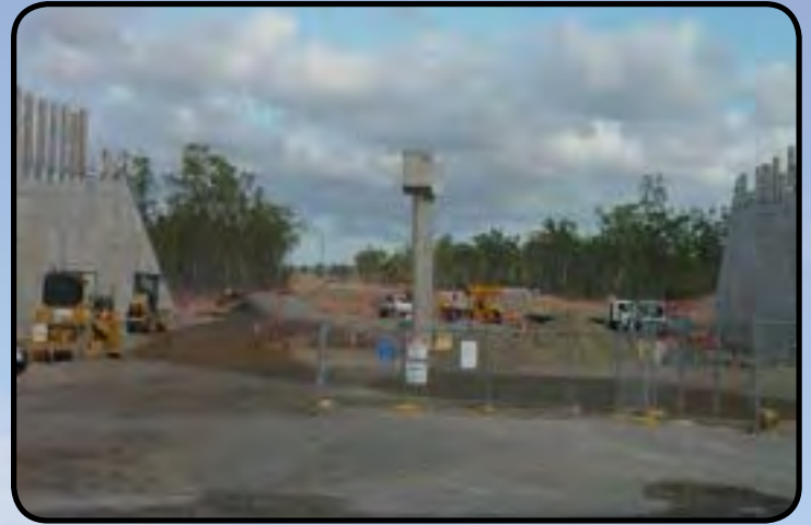
Blade walls complete on Shaw Road overpass
