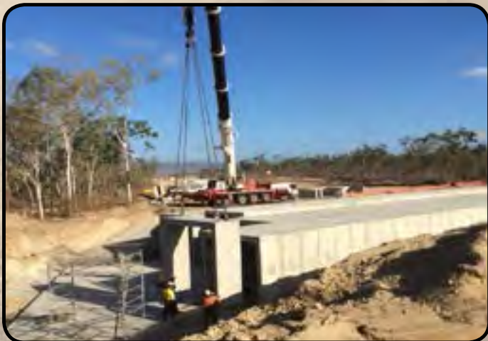
Constructing culverts on the alignment
