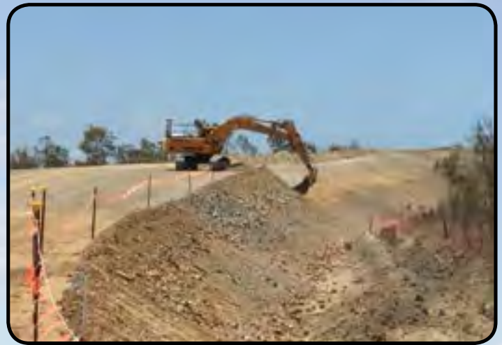
Placing embankment material
