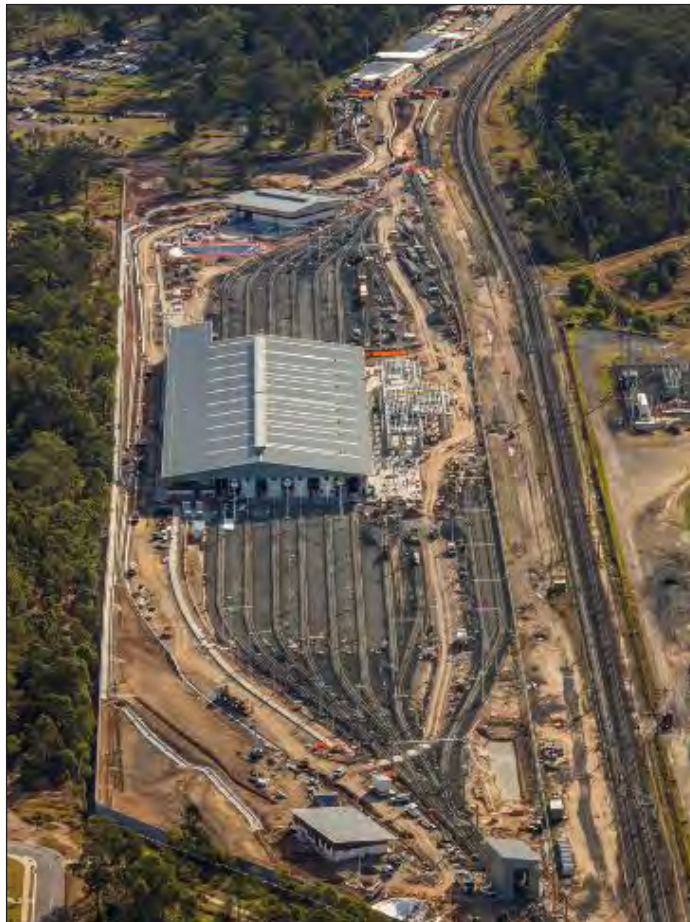
Wulkuraka Maintenance facility and outlying stabling yards, photo courtesy of TMR.
