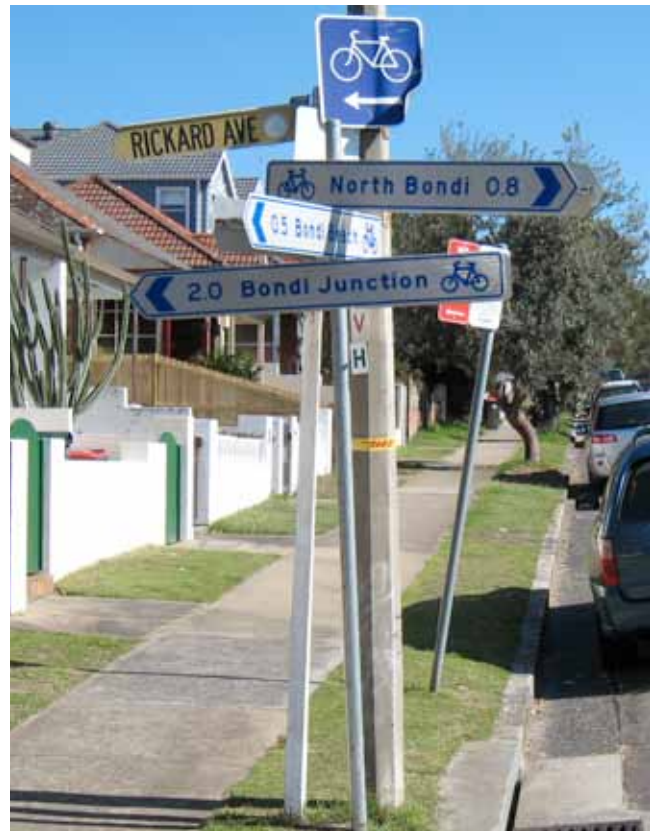
Photo 16: Poor practice example of cycle network signage in an urban environment. This four-way intersection has cycle routes on three legs. The cycle route signage is poorly mounted with double, back to back signs for each cycle leg. These are centre mounted on a new steel pole. The street sign has its own timber pole. The badly faded and unreadable community sign and the blue cycle route sign above it are redundant and should be removed. The damage sustained by the blue marker, points to the eventual fate of this sign group. Bondi NSW.
