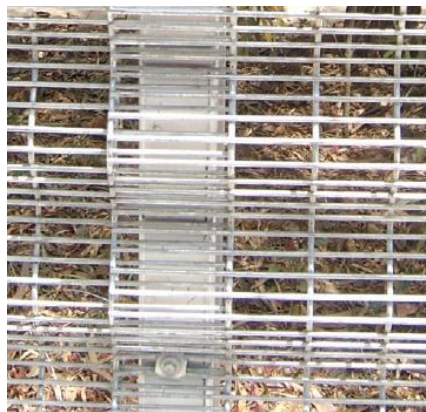
Figure 1 - Closely spaced mesh fencing
