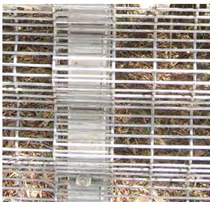
**Figure 1 - Closely spaced mesh fencing**
