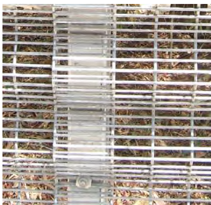
Figure 1 - Closely spaced mesh fencing
