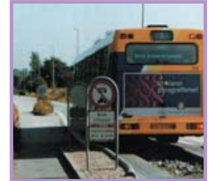
Figure C3-3 This bus gate provides connectivity for pedestrians and cyclists, but not cars
