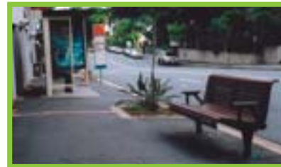
Figure D1-21 Bus stops and shelters can reduce sightlines and narrow the effective path width
