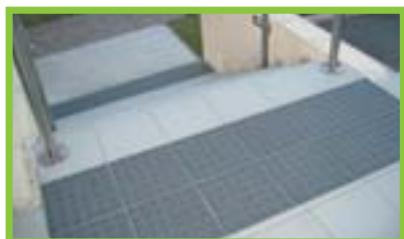
Figure D1-2 Tactile ground surface indicators (TGSIs) are essential near hazards
