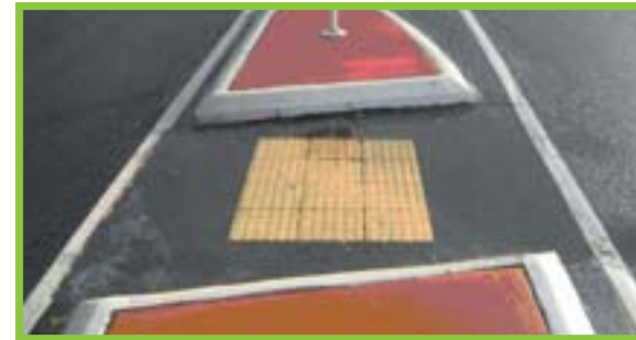
Figure D1-6 Example of a pedestrian refuge (note the insufficient width of the tactile indicator)
