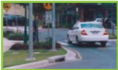
Figure D1-8 Ensure that pedestrians are clearly visible to motorists at pedestrian crossings. (Note how pedestrian is partially obscured by vegetation and utility poles in this photograph.)
