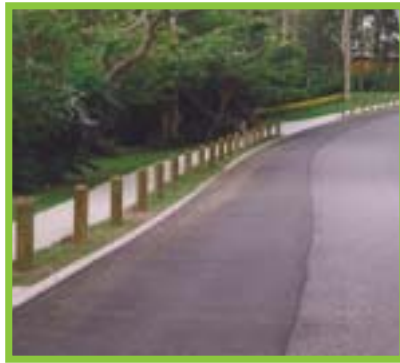
Figure D2-1 Measures may be needed to ensure that accessibility is maintained (e.g. bollards protecting pedestrians from parked vehicles)
