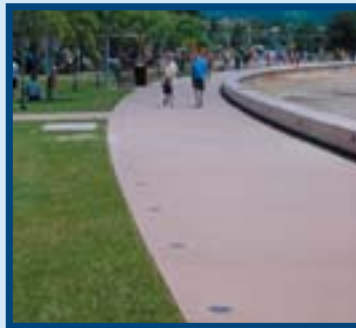
Figure D3-4 Cairns Esplanade. The top photograph shows a surface selected to reduce glare. The bottom photograph shows joints designed to minimise cracking.
