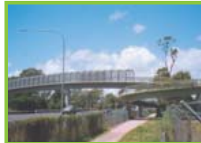
Figure D3-5 Overhead cages protect passing vehicles (and other users) from the risk of projectiles being thrown from the overpass
