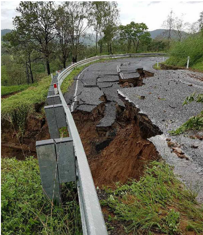
Severe landslips closed the Sarina Range on Marlborough-Sarina Road.
