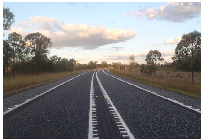
Wide centreline treatment with audio tactile line marking.
