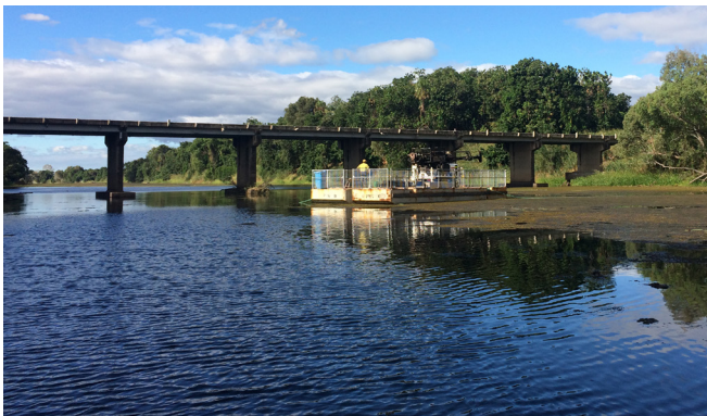
Barge drilling at Haughton River bridge.
