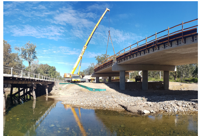
The new bridge at Boundary Creek under construction in June 2017 as part of the Peak Downs Highway Timber Bridges Replacement Project.
