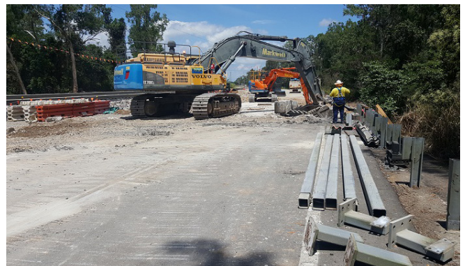
Existing decking being removed from the Arnot Creek bridge.
