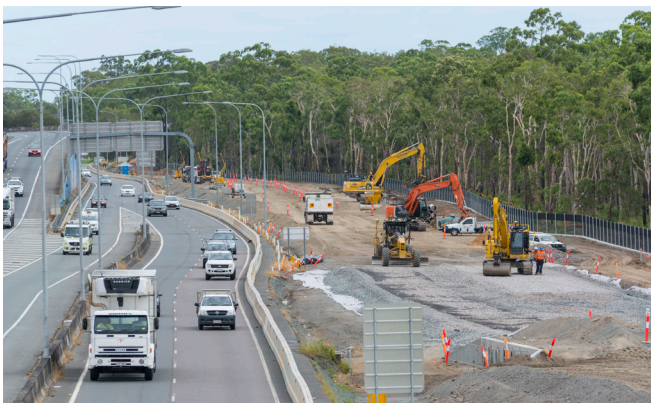
Gateway Upgrade North – Deagon Deviation widening.
