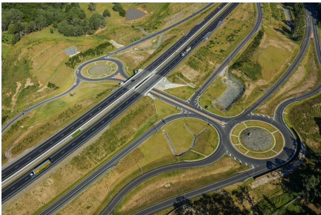
Aerial view of the completed Cooroy to Curra (Section A) northern interchange. Photo by Above Photography.
