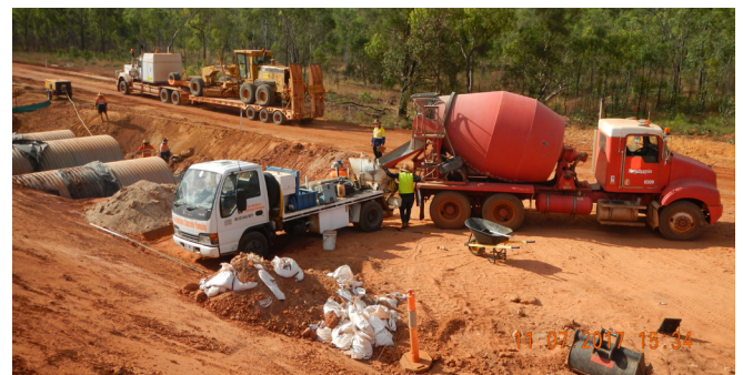
Construction on the Peninsula Developmental Road, Archer to Wolverton.
