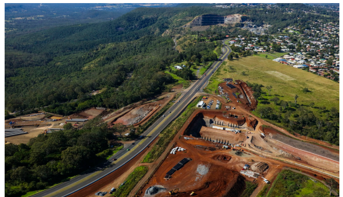
Construction of the New England Highway twin arch bridges.
