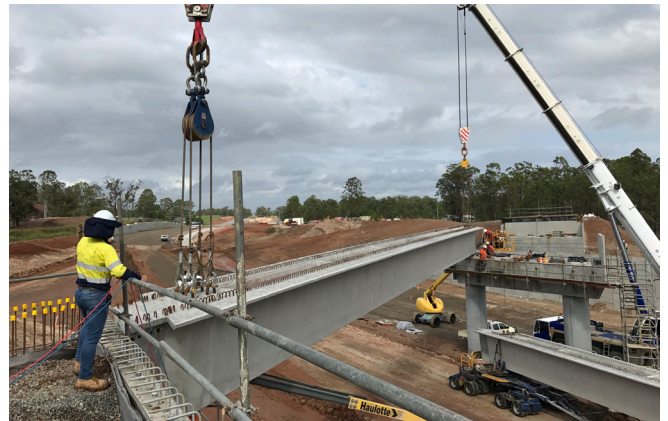
Girder placement at Tinana Interchange.
