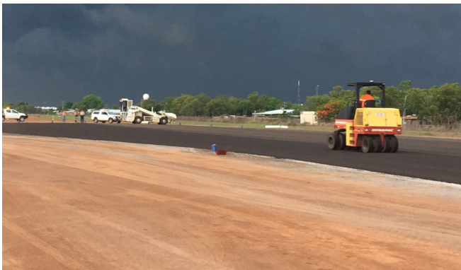
Our crews worked to ensure the remote community wasn't isolated.
