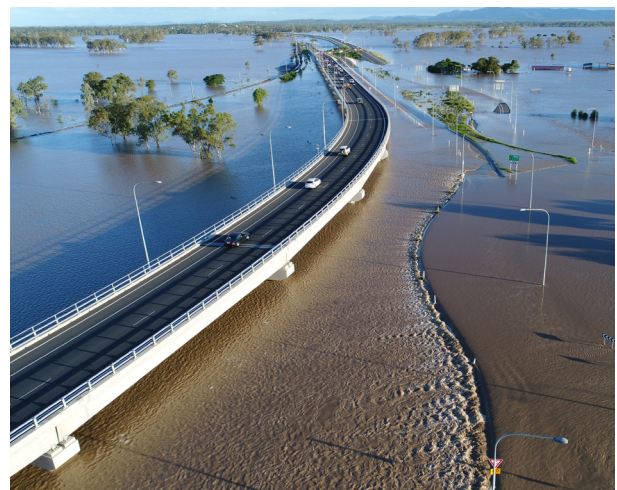
Yeppen Floodplain Crossing following Ex-Tropical Cyclone Debbie.
