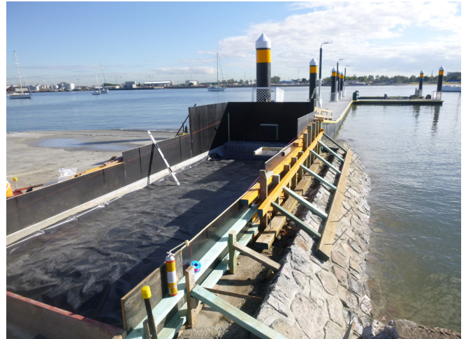
Colmslie boat ramp construction.
