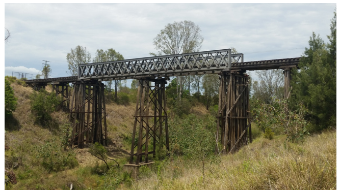
Lockyer Creek bridge will no longer serve as a rail bridge but be part of a Brisbane Valley Rail Trail.
