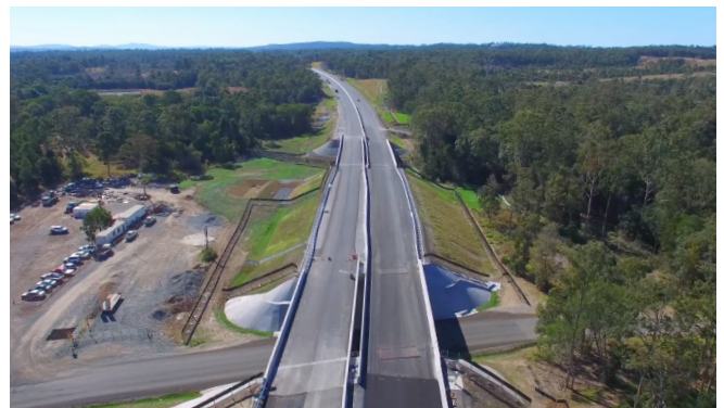
New Bruce Highway bridges over Tandur Road looking north.
