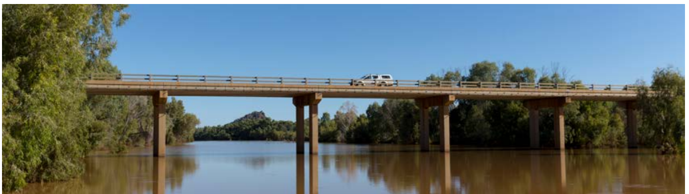
Cloncurry River Bridge, Cloncurry Shire
