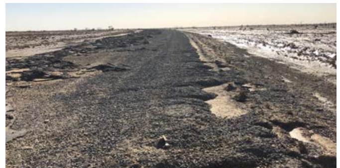
Flinders Highway in between Richmond and Julia Creek, damaged road from flooding during February 2019.
