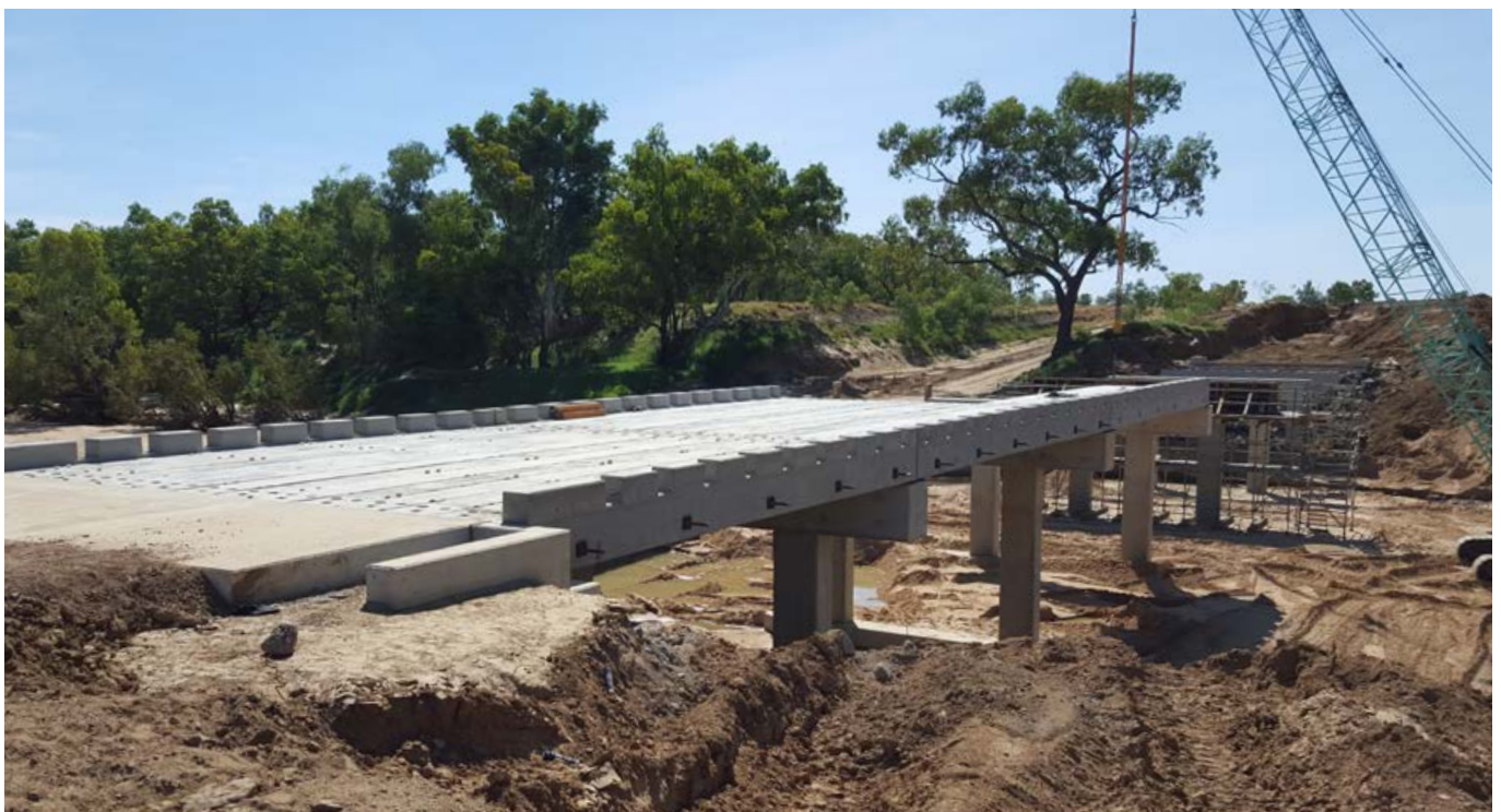
Construction of Hulberts Bridge, Richmond
