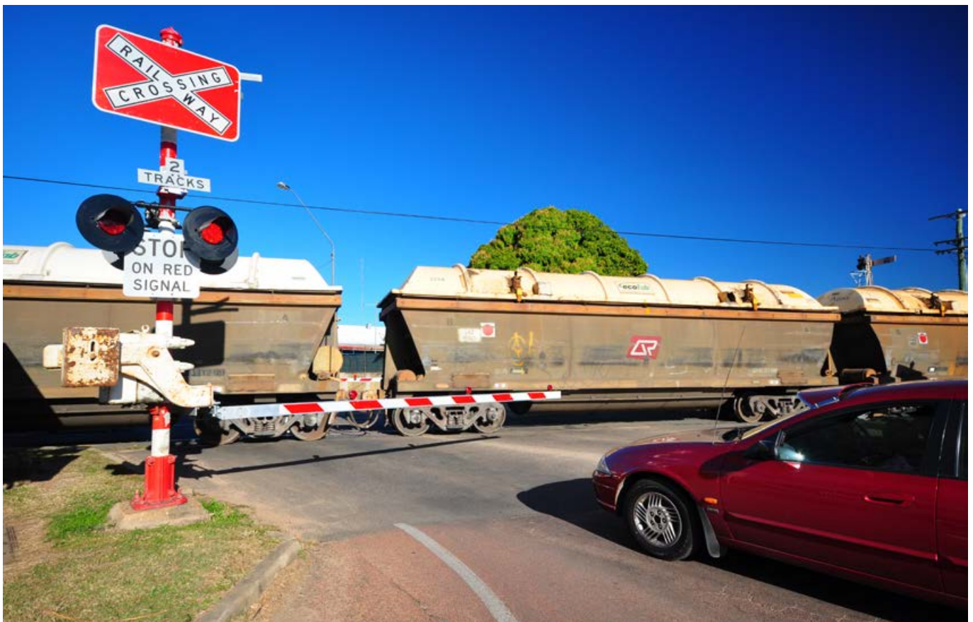
Open level crossing, Charters Towers
