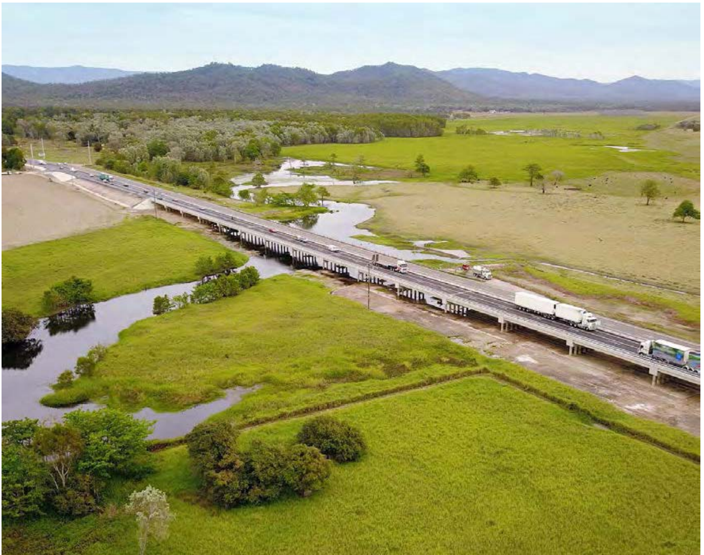
Cattle Creek Bridge on the Bruce Highway, south of Ingham, as part of the Cattle and Frances Creek Upgrade Project.
