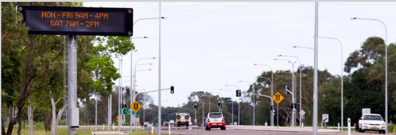
Variable message sign, Bruce Highway
