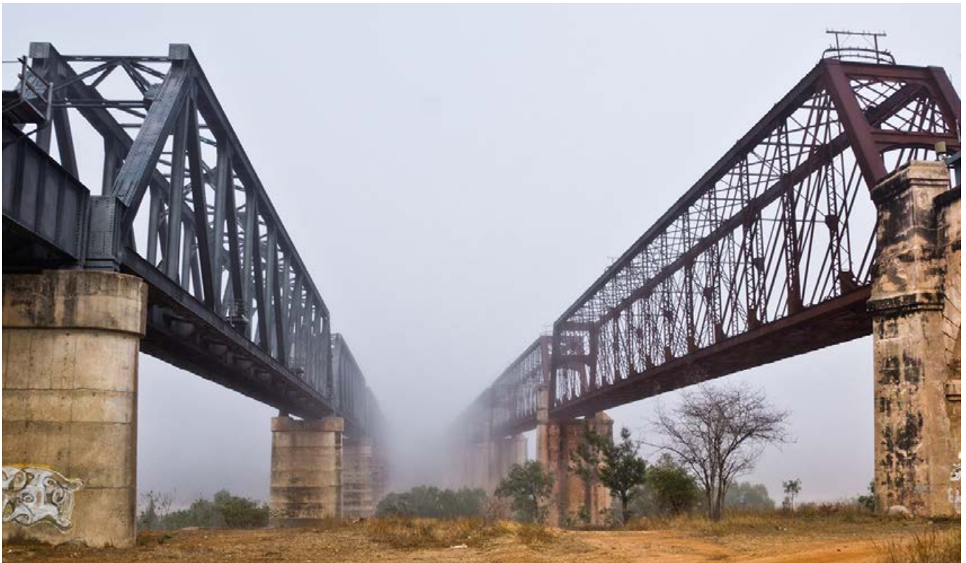
The Macrossan Rail Bridge (the bridge to the left), Charters Towers, is a key component of the supply chain in North West and Northern Queensland to support opportunities in mining, tourism, agriculture and industry. The Burdekin River Rail Bridge to the right is heritage listed and is decommissioned.
