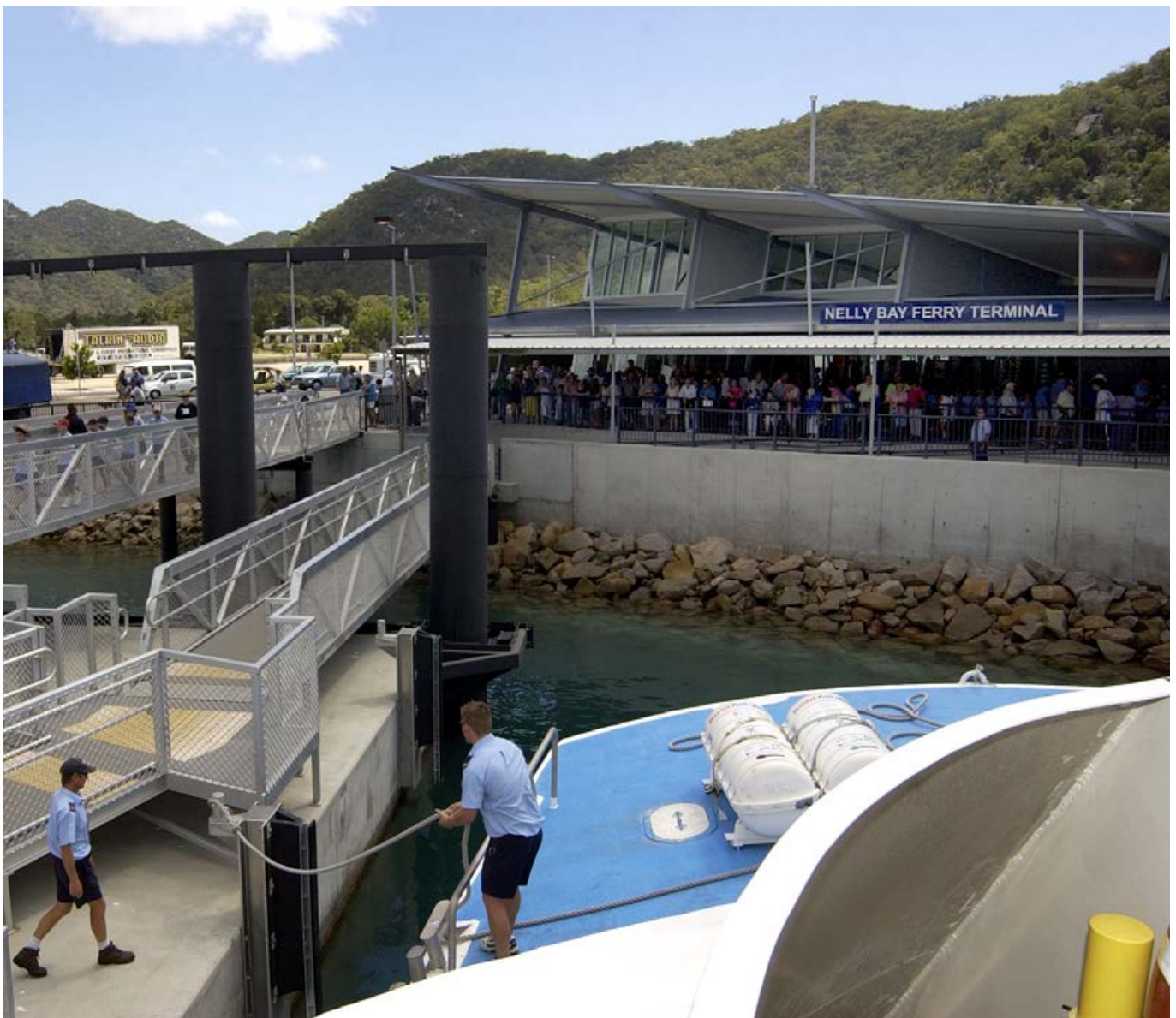
Nelly Bay Ferry Terminal, Magnetic Island
