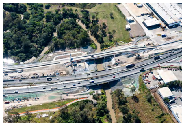
Ipswich Motorway Upgrade – Rocklea to Darra (Stage 1) project: Construction of new motorway bridges over Oxley Creek floodplain (Photo credit: R2D Aerials Press 39).
