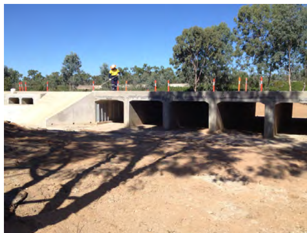
An example of a fish passage delivered at Puddler Creek, west of Charters Towers.
