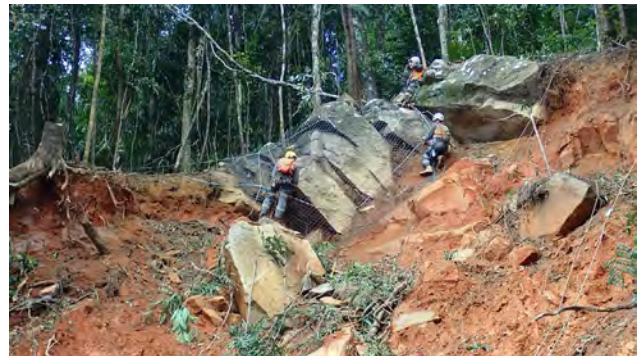
Geotechnical contractors removing unstable boulders on Mount Spec Road, Paluma, reducing the risk of further landslips after natural disasters.
