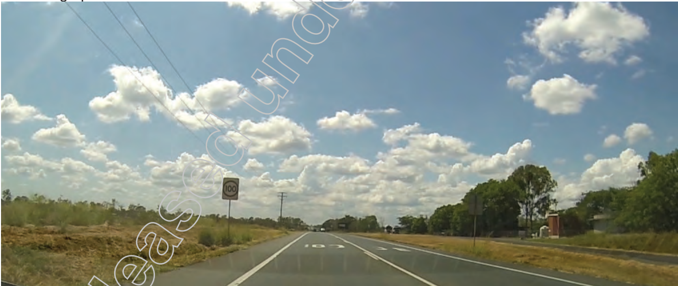
Photograph 2.2 Eastbound Section C 80km/h to Section B 100km/h
