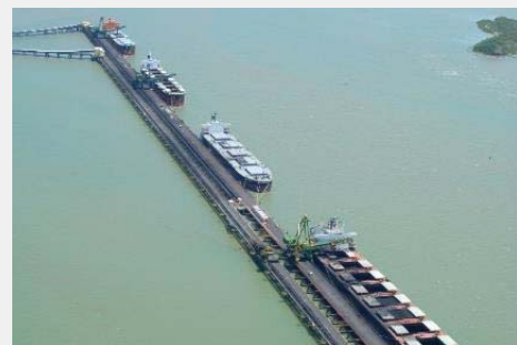
Case study 3 – Four berths being serviced by three shiploaders at the RGTCT.
