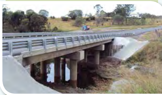
Geramanbulyan Bridge Upgrade.
