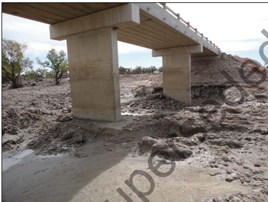
**Figure 2.1A: Pier and abutment scour due to inadequate design**
