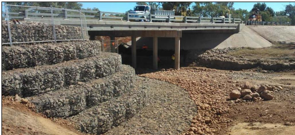
**Figure 3.1.1: Various protection measures used in repair works**
