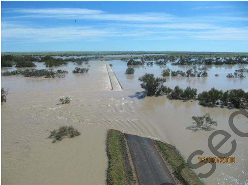
**Figure 1.4.3A: Overtopping of the Burke and Wills bridge is an example of vertical contraction scour**
