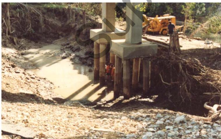
**Figure 1.5.1A: Local scour damage at piles on the Logan River**
