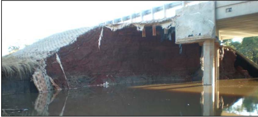
**Figure 1.5.3A: Scour of abutment protection**
