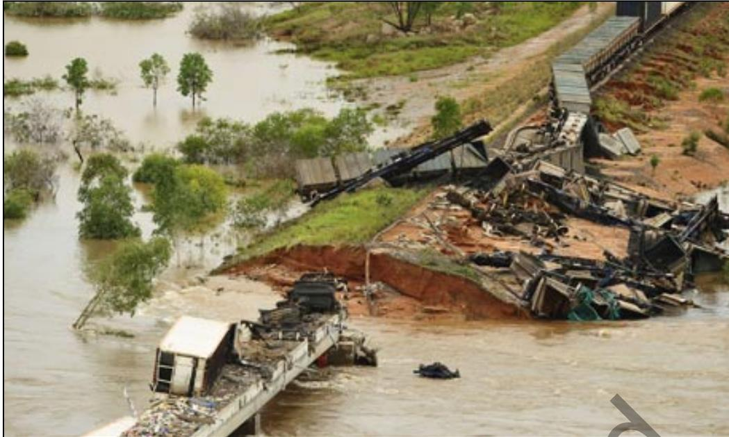
**Figure 1.1: Derailment and railway embankment failure during Cyclone Grant on Adelaide to Darwin railway (picture: Michael Franchi)**
