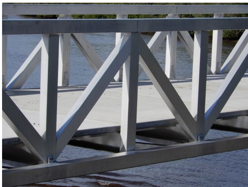
Figure 15.2.1 – Eudlo Creek bridge (under construction) showing precast deck slabs
