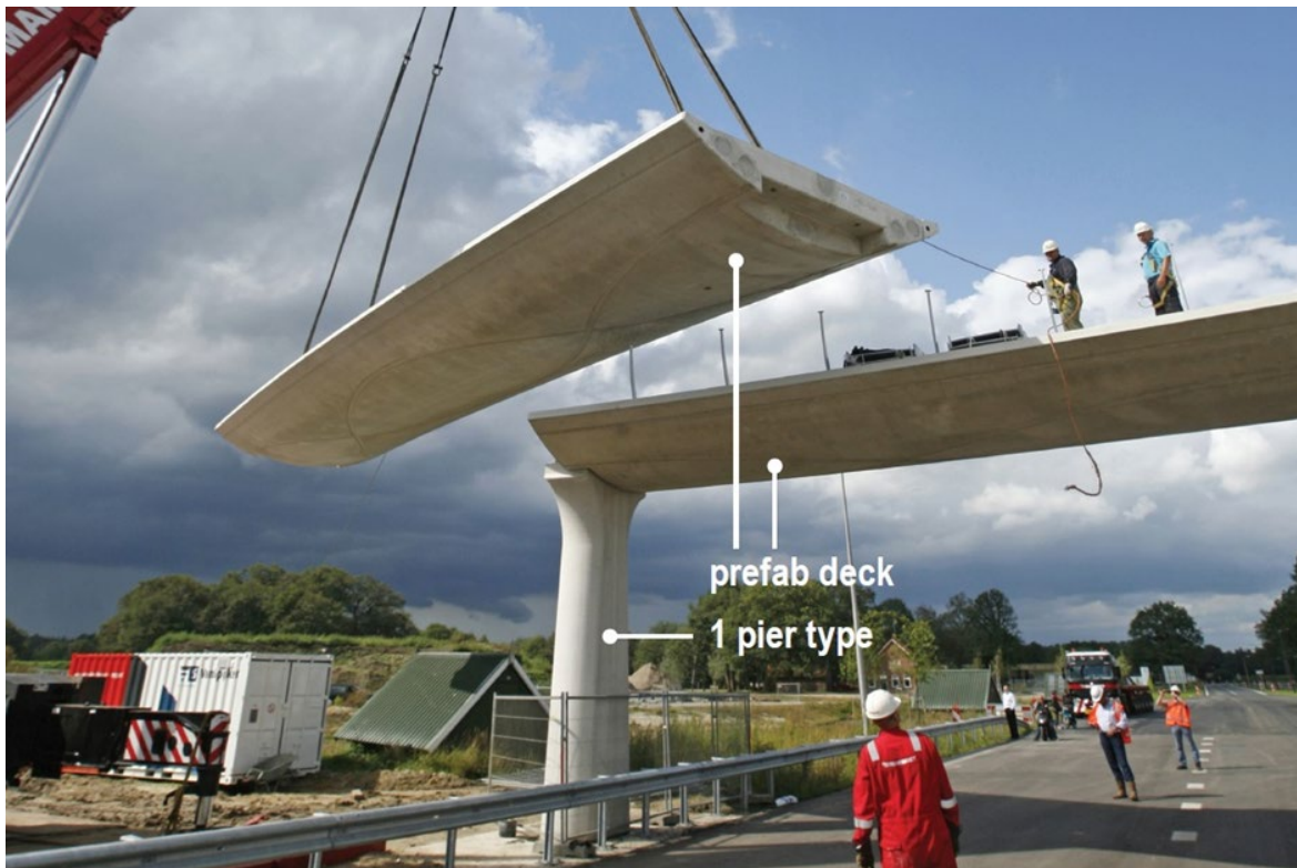
Figure 25 – Auke Vleerstraat bridge at Enschede (The Netherlands), under construction
