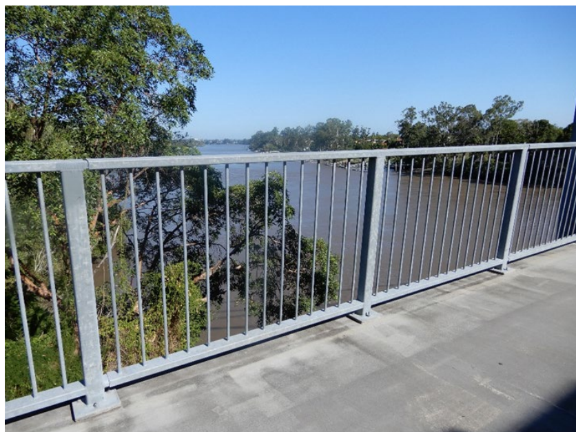
Figure 20.1(c) – Balustrade at Jack Pesch Bridge, Indooroopilly
