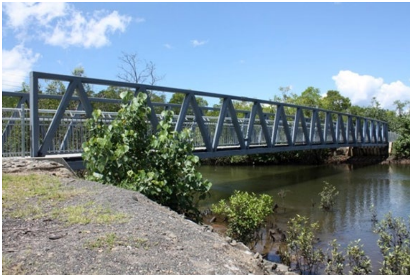
Figure 14.6.1 – Bridge at Moody Creek, Cairns
