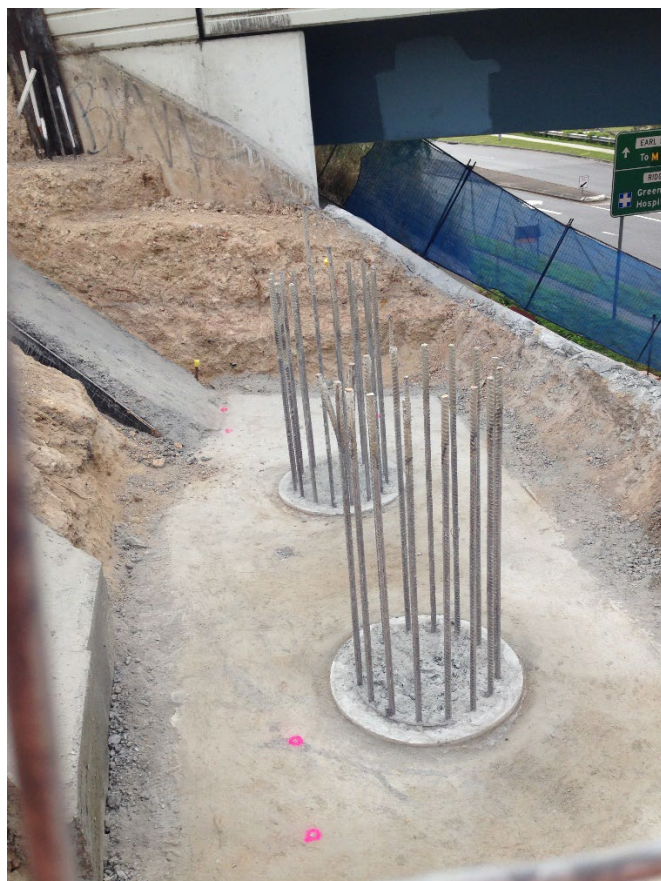
Figure 23.4 – 900 diameter piles for Lewisham Street cycle bridge on V1, Brisbane
