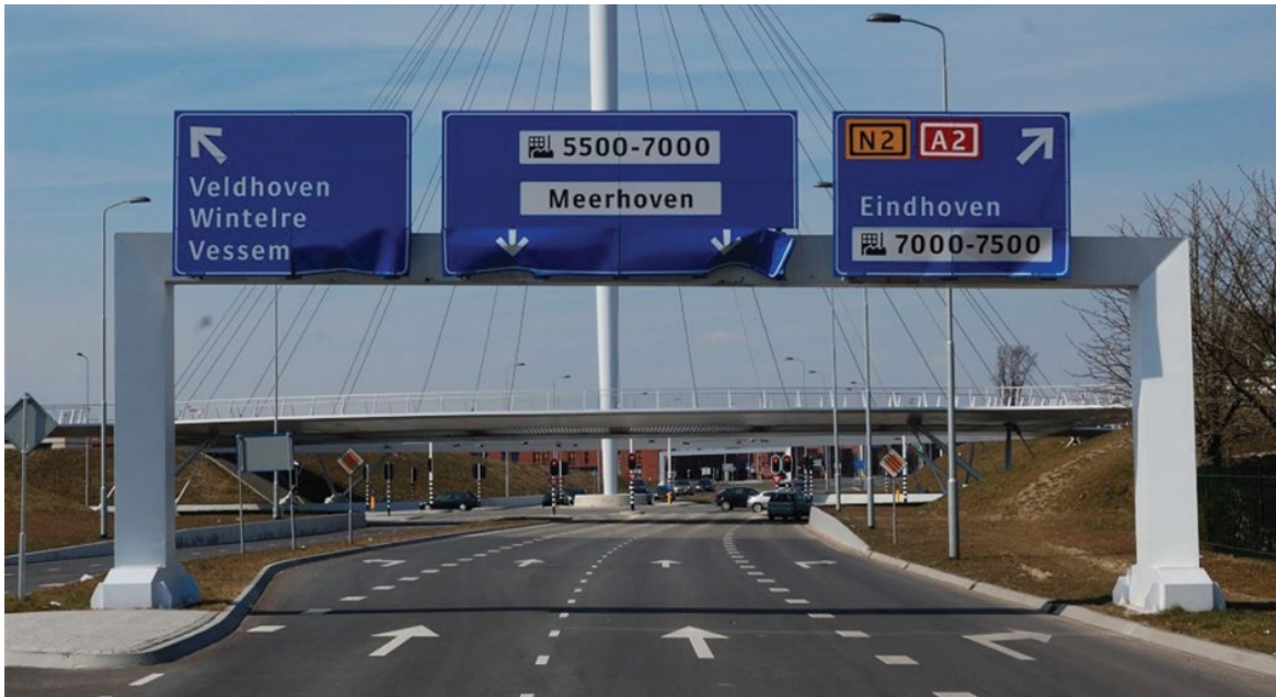
Figure 11.2(b) – Combined stop barrier and signage at the Hovenring
