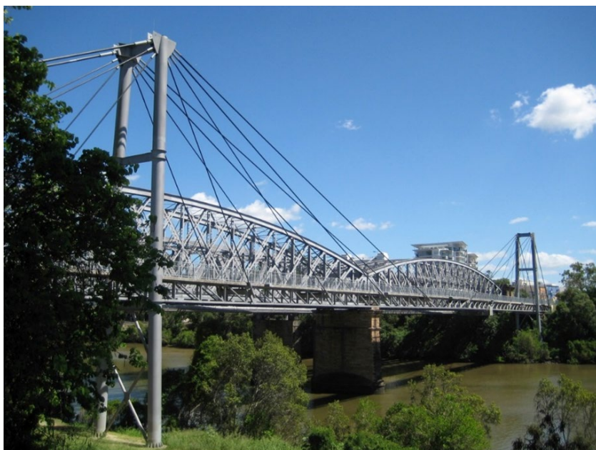
Figure 14.8 – Jack Pesch cable stayed bridge at Indooroopilly
