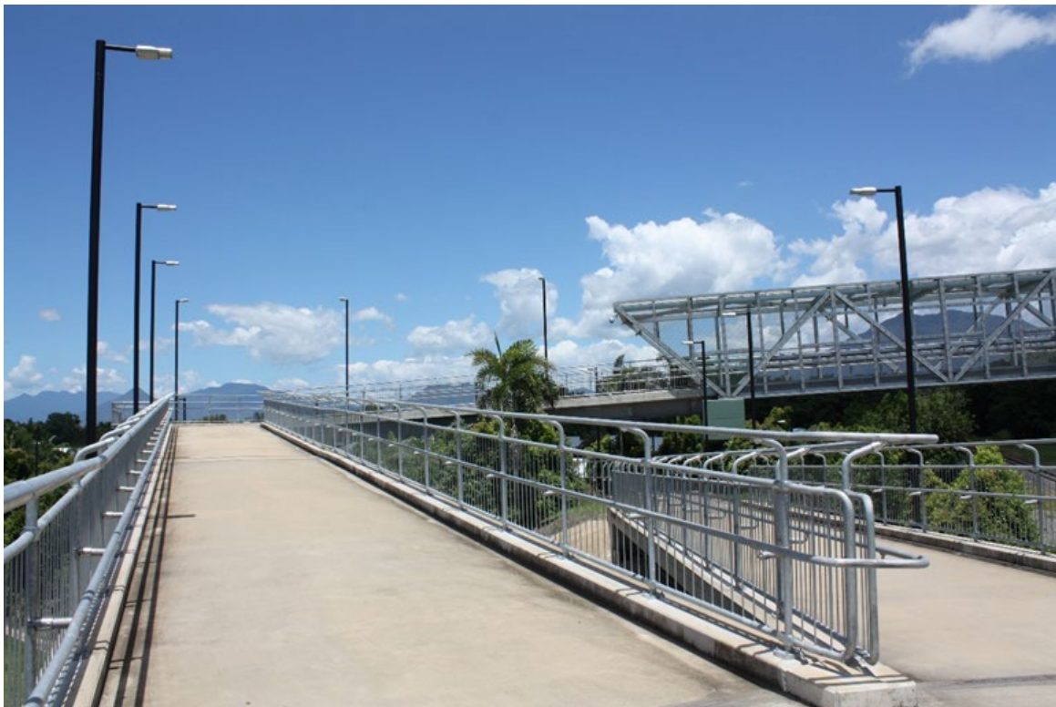
Figure 20.1(e) – Installed proprietary barrier for the Cairns Connect bridge
