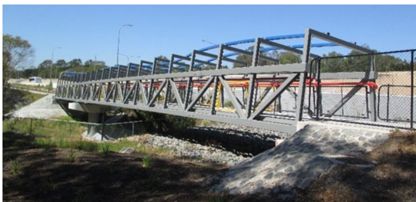
Figure 14.6.2(a) – Ekibin Creek cycle bridge
