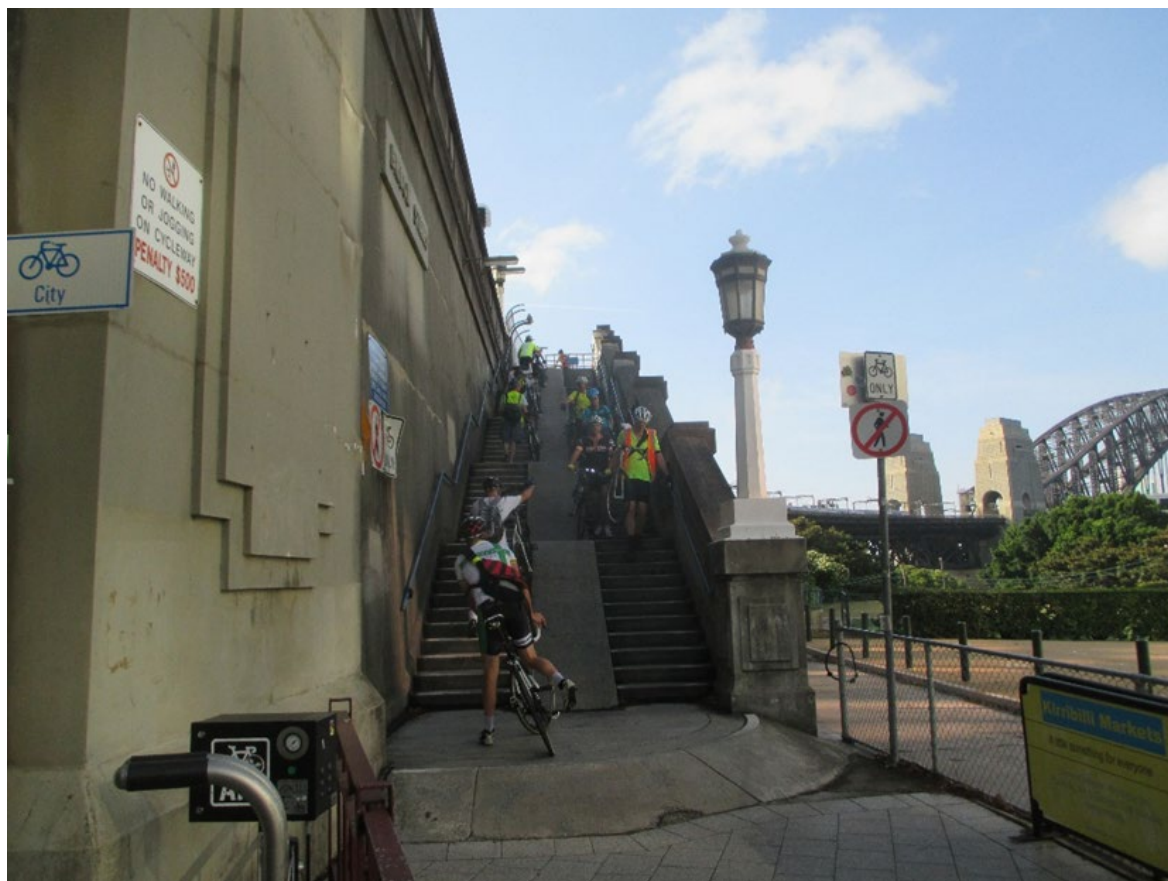
Figure 12.3(c) – Stairs only access to Sydney Harbour Bridge cycleway
