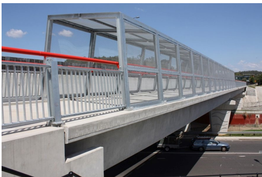
Figure 22(b) – Lewisham Street cycle bridge
