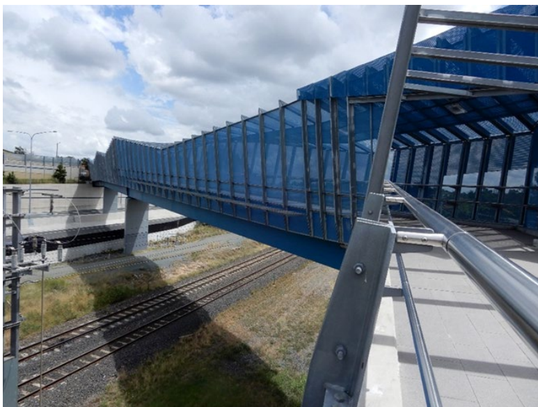
Figure 2.2(b) – Goodna State School shared use bridge over the Ipswich rail line and Ipswich Road.
