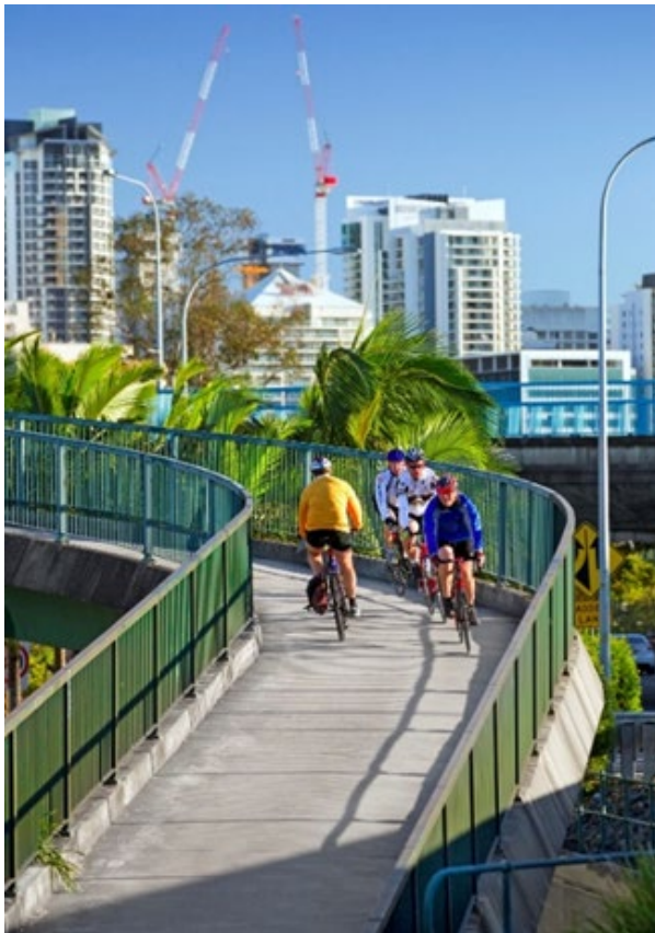
Figure 14.3.3(c) – Stanley Street on-ramp bridge
