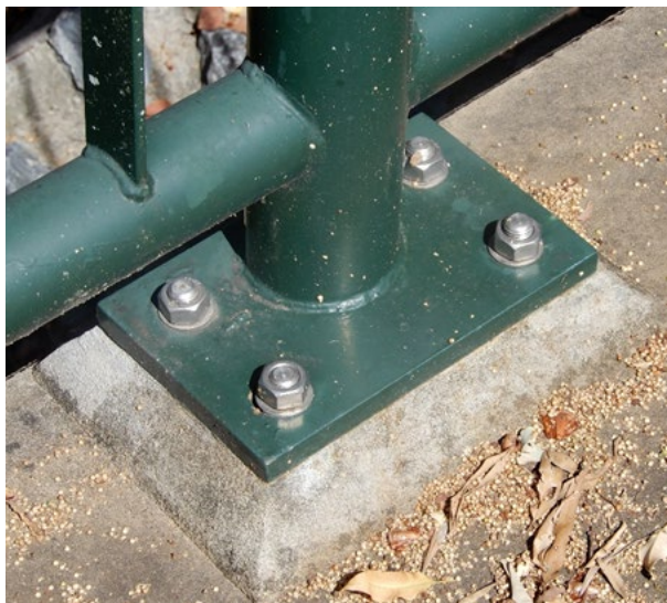
Figure 13.3(d) – Stainless steel hold down bolts
