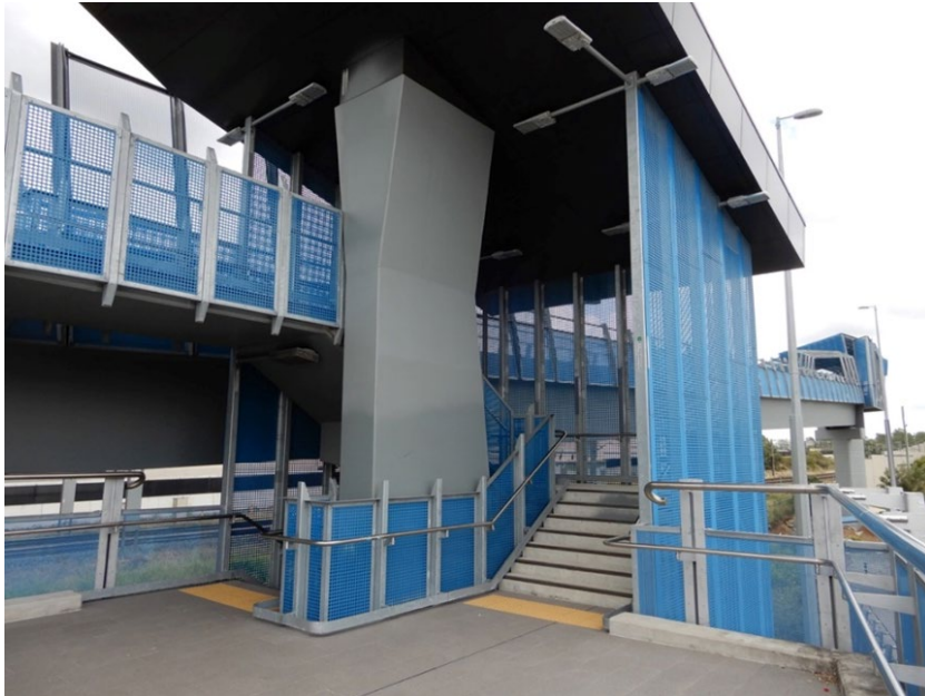
Figure 12.3(a) – Access stairs at Goodna State School bridge
