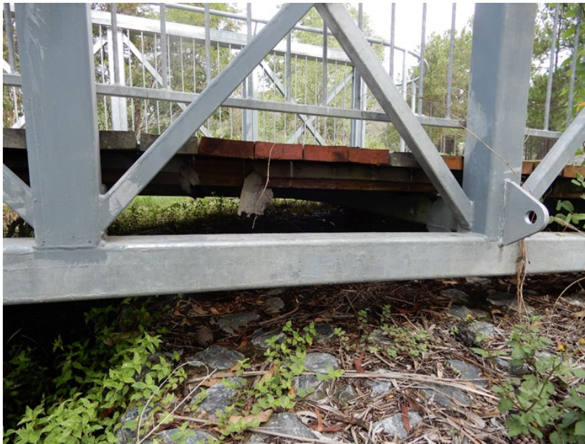
Figure 15.6(b) – Timber deck on bridge over Bulimba Creek (Craig Street, Wishart)
