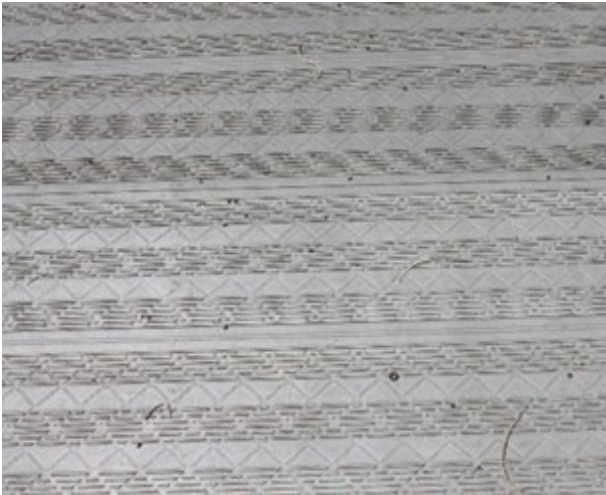
Figure 15.3(b) – Textured deck surface on bridge at Aeroglen
