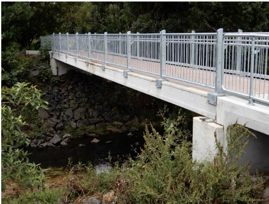
Figure 14.5.2 – Maleny Trail shared use bridge
