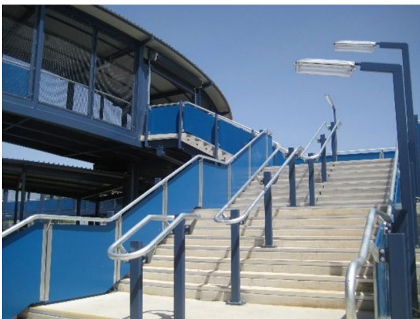
Figure 12.3(b) – Stairway access for students at Redcliffe State High School
