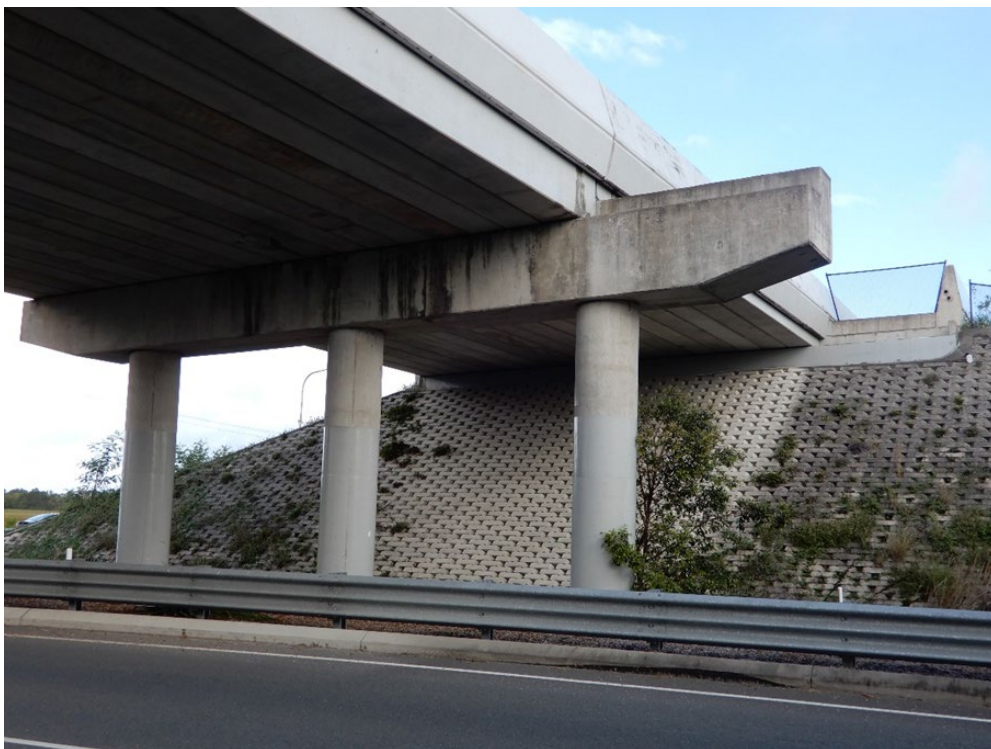
Figure 6.2 – Widened substructure to enable future erection of superstructure
