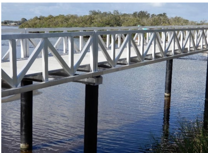
Figure 14.6.3(b) – Eudlo Creek shared use bridge (during construction)
