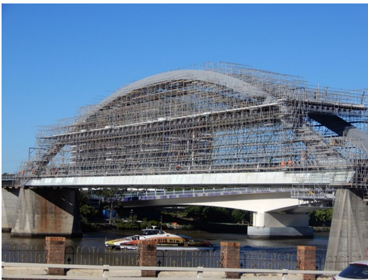
Figure 24 – Maintenance work at Merivale Rail bridge
