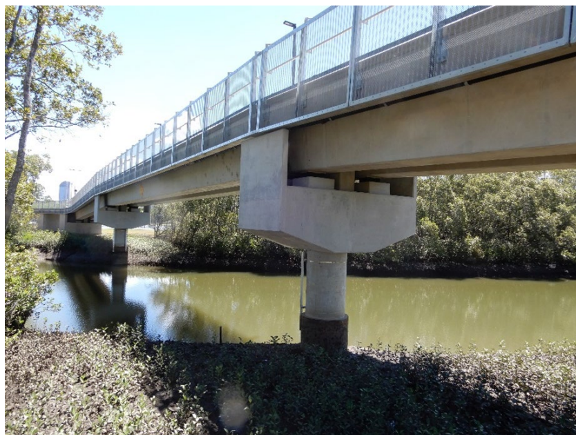
Figure 2.2(c) – Shared use waterway crossing
