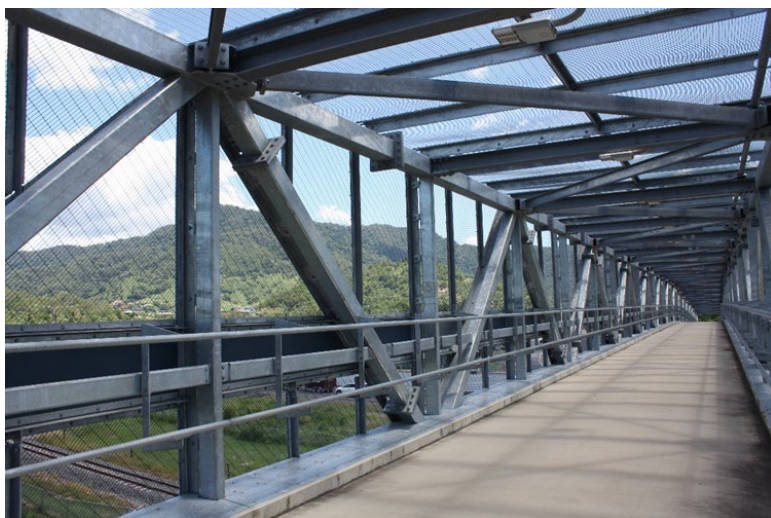
Figure 13.3(b) – Anderson Road bridge, Cairns
