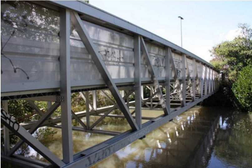
Figure 15.3(a) – Bridge over Saltwater Creek at Aeroglen, Cairns
