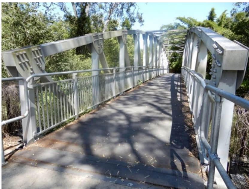
Figure 14.6.3(a) – Jindalee Park bridge
