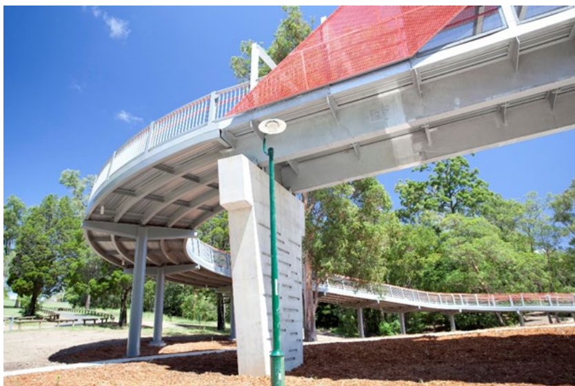
Figure 13.1 – Toowong Crossing shared use bridge
