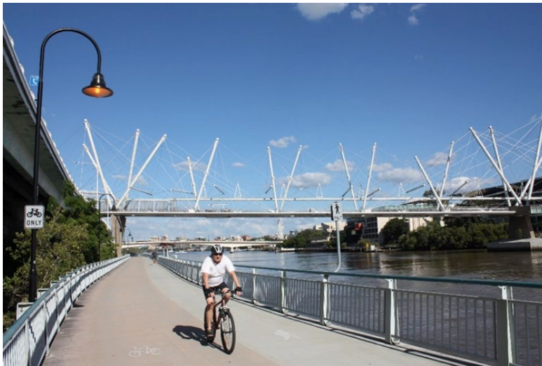
Figure 2.2(a) – Kurilpa shared use bridge over the Brisbane River, viewed from the Bicentennial shared use bikeway and boardwalk
