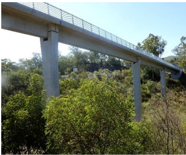
Figure 14.3.2(a) – Moggill Road cycle bridge
