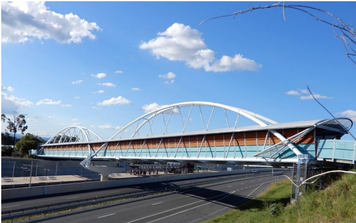
Figure 14.7(a) – Springfield shared use bridge
