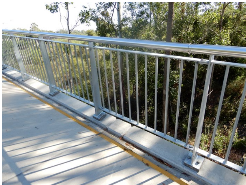
Figure 20.1(b) – Bespoke balustrade at Moggill Road cycle bridge
