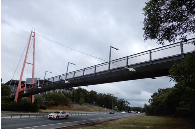
Figure 5(a) – Griffith University shared use bridge, Gold Coast
