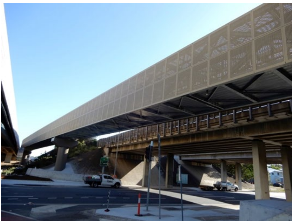
Figure 14.6.2(b) – Juliette Street cycle bridge
