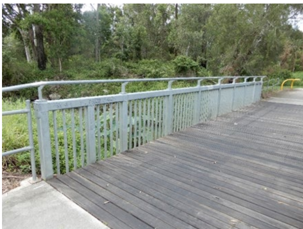
Figure 15.6(a) – Timber deck on bridge over Bulimba Creek (Ditmas Street, Wishart)
