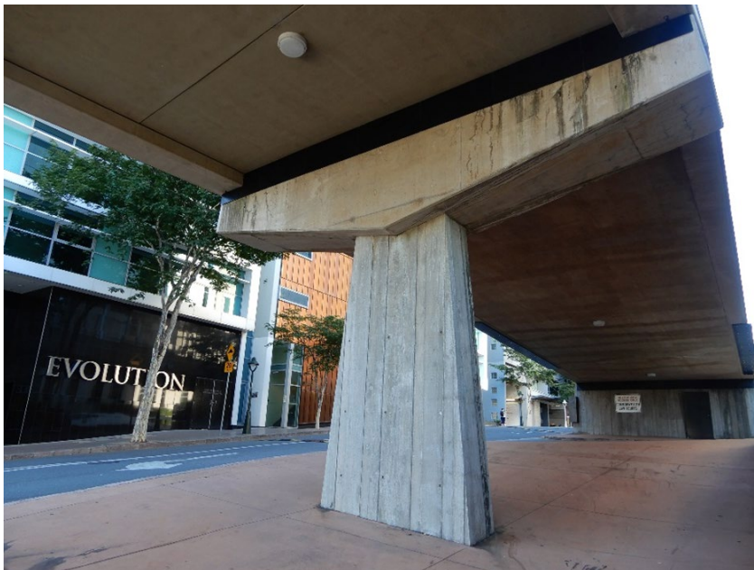
Figure 5(c) – Kurilpa Bridge pier, Tank Street, Brisbane
