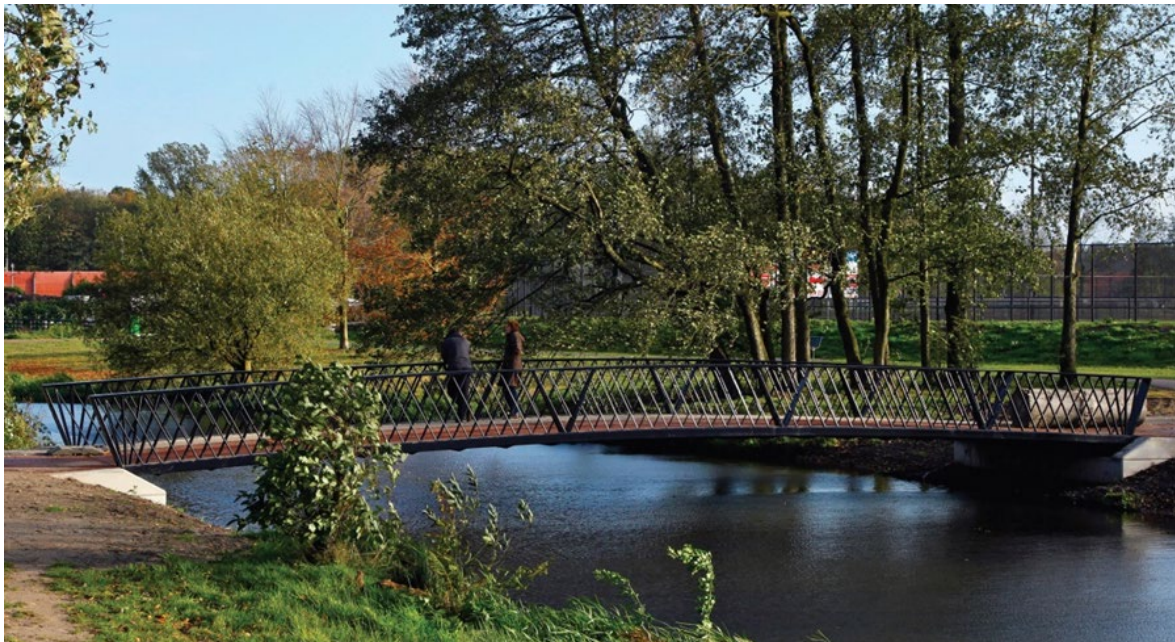
Figure 20.1(a) – Lattice truss balustrade
