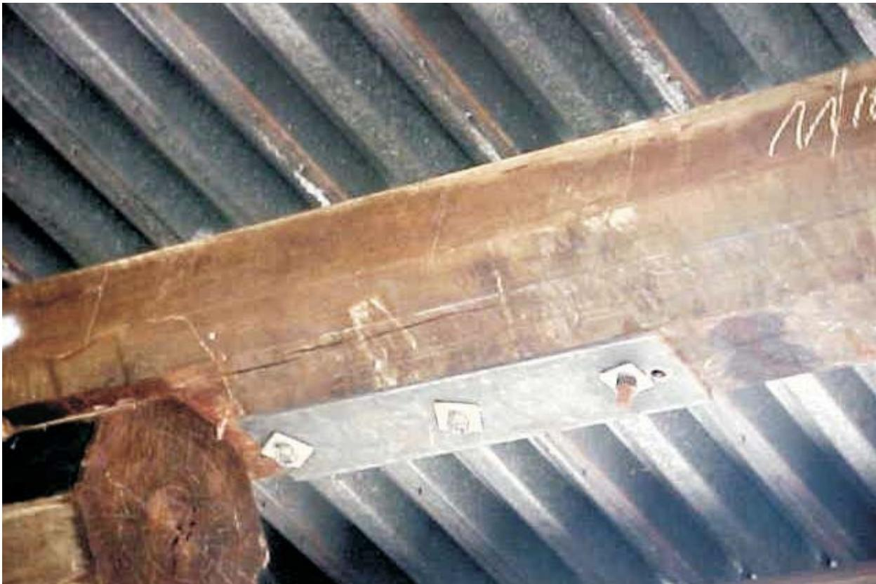
Figure 4.6(c) - Notch Cracking
