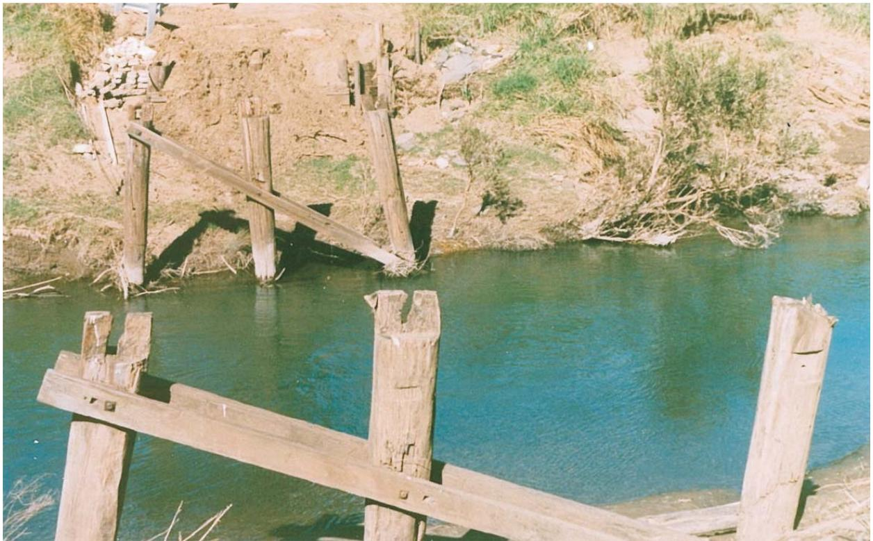
Pier pile failure at top
