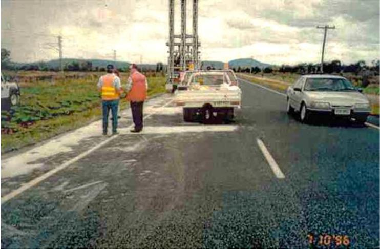
**Figure 4.9.7.7(d) – Example of lime injection pods**
