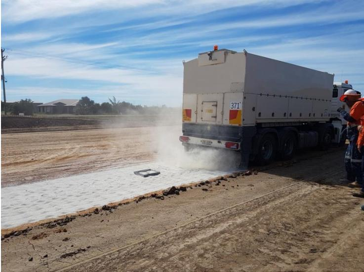
**Figure 4.9.7.6(b) – Slaking of quicklime**
