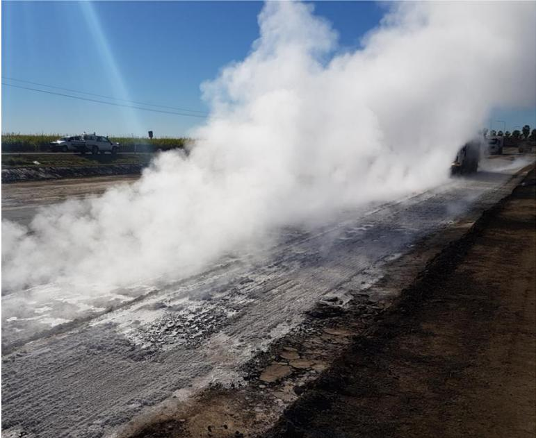
**Figure 4.9.7.6(d) – Steam cloud generated during slaking of lime**
