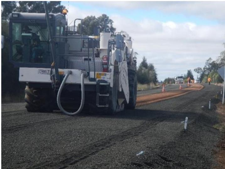
**Figure 4.9.8.6.1(c) – Grading to receive additive (before spreading or addition of any stabilising agent)**
