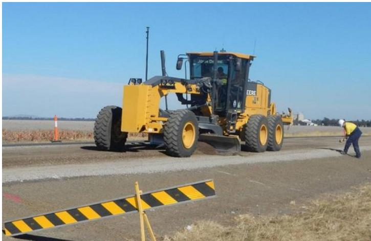
**Figure 4.9.8.6.1(j) – Target depth needs to account for the bulked height above finish surface level**
