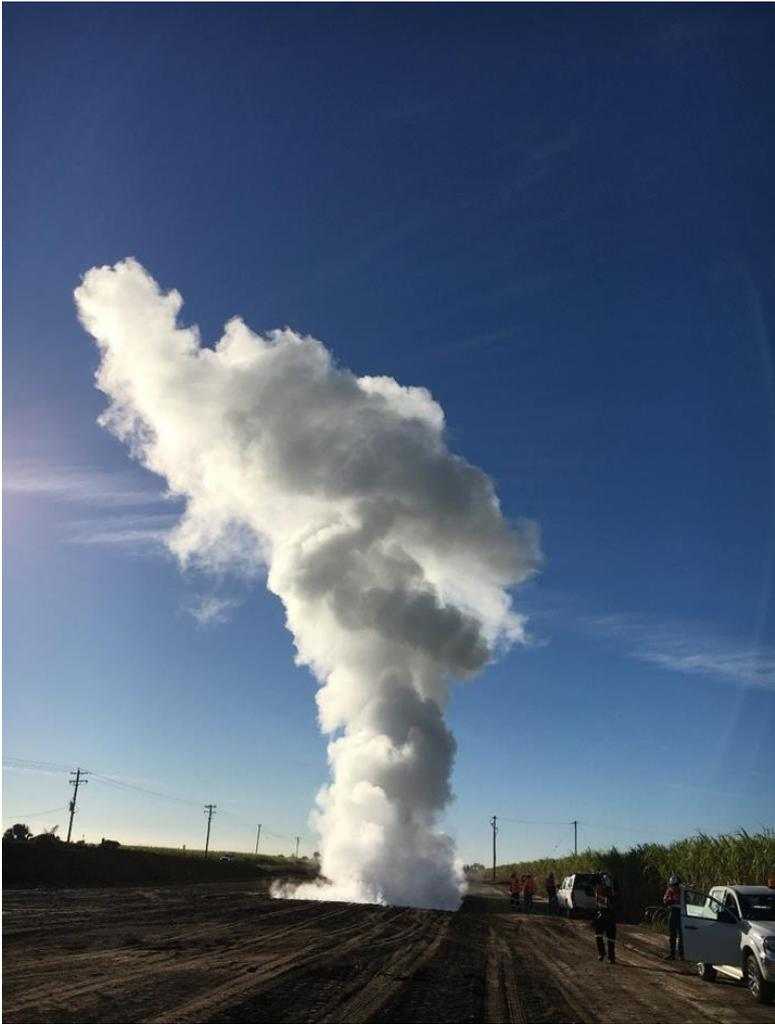
**Figure 4.9.7.6(e) – Lime stabilisation of an expansive-soil subgrade in the outer region of a pavement**
