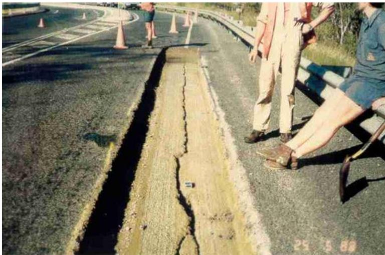
**Figure 4.9.7.1.2(c) – Typical shrinkage cracking of expansive soils**
