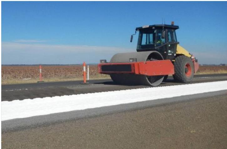
**Figure 4.9.8.6.1(i) – Grading / shaping prior to the final foamed bitumen incorporation pass**
