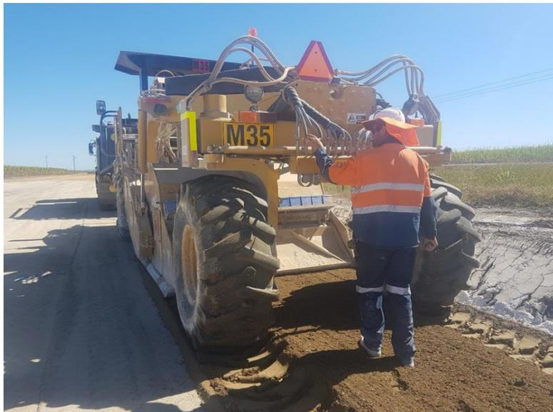
As noted in Section 4.9.7.5, it is essential, where quicklime is used, the dosage used in the field is adjusted to take account of the impurities present in the quicklime used and the fact laboratory testing was undertaken using hydrated lime.
