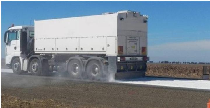
**Figure 4.9.8.6.1(f) – Spreadrate test in operation**
