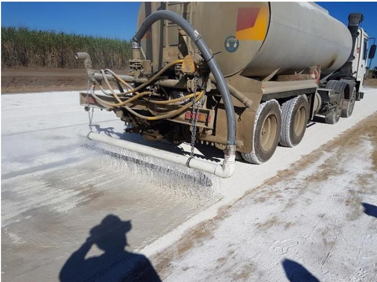
**Figure 4.9.7.6(c) – Slaking of quicklime**
