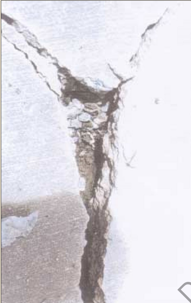
Close-up of typical crack in apron slab.
