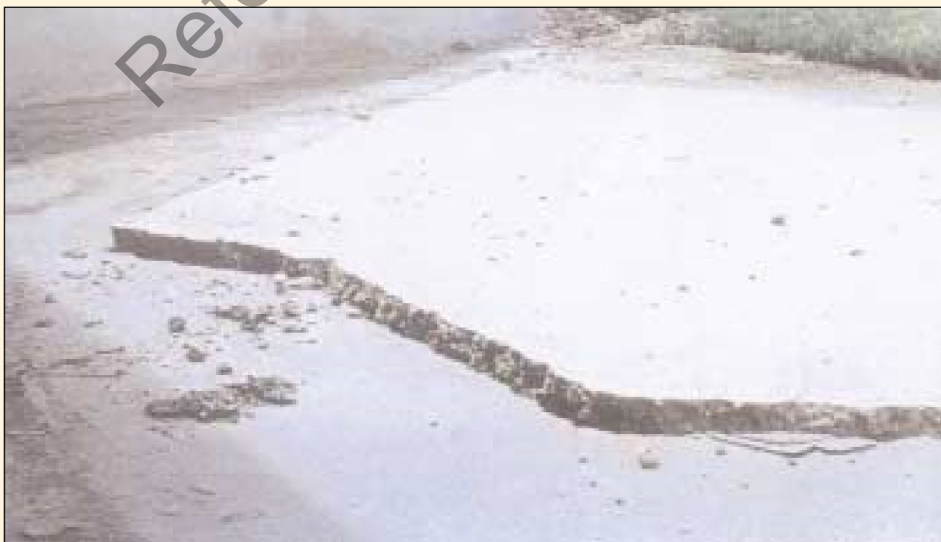
Typical apron slab crack near the wing wall slab. Note the vertical displacement across the break, and the rise of the apron slab relative to the wing wall slab.
