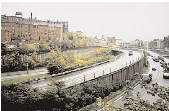
Split carriageways in urban setting
