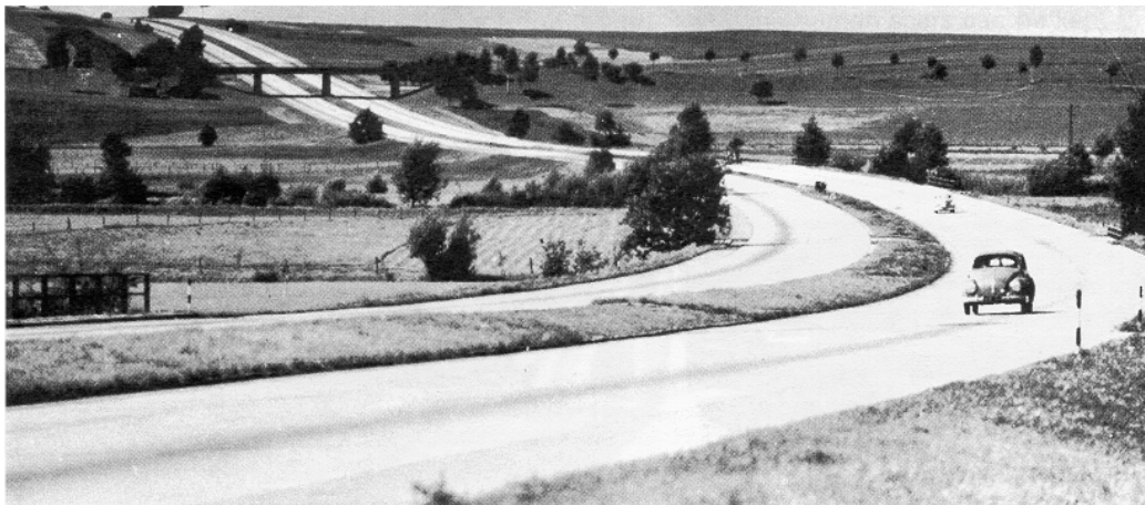
A road well fitted to the terrain. This has been achieved by the use of continuous liberal curves.
