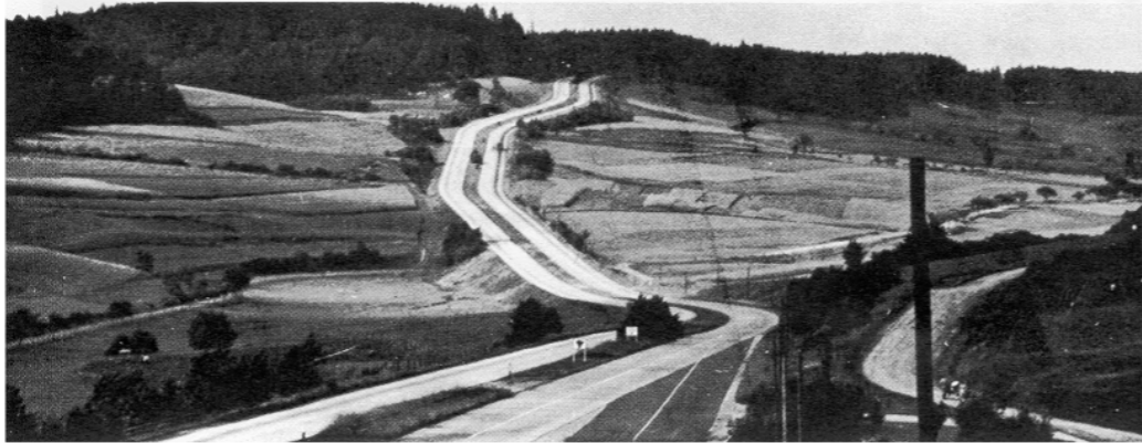
A road which is not well fitted to the terrain. The use of long tangent, short curve design creates this lack of relationship with the generally gently rolling countryside.
