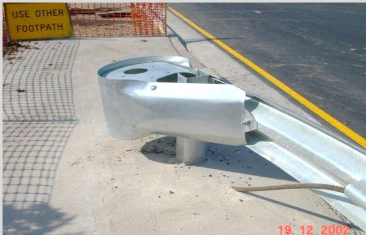
The first photo (above) depicts frangible elements, slip base posts and tension cables, buried by concrete / median / kerbing level. This prevents the system from functioning and eliminates the intended safety benefits.
